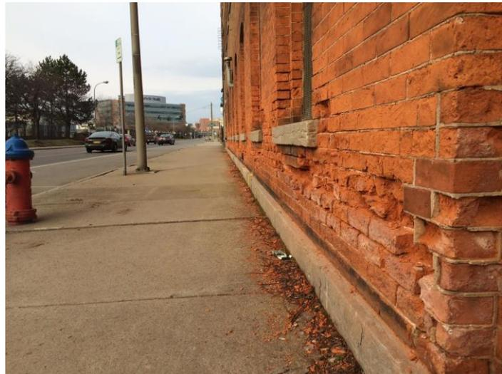
*A cocktail of traffic pollutants including rock salt and reactive chemicals like nitrogen oxides (NOX) is causing the brick on this privately owned building on Elm Street in Buffalo to decompose prematurely.*
