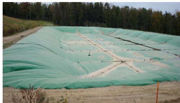
Figure 1. Impermeable HDPE cover installed on an existing earthen dairy manure storage in New York State
