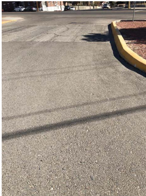
Figure D-2. Sidewalk missing on one side of Upson Dr.
