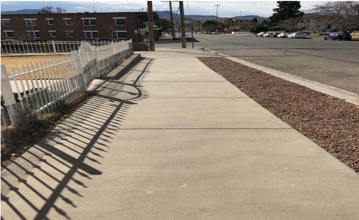
Figure B-2. Sidewalk in general good condition, Yandell Dr.
