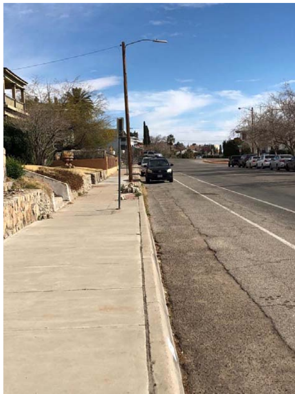
Figure A-2. Sidewalk in general good condition on Prospect St.
