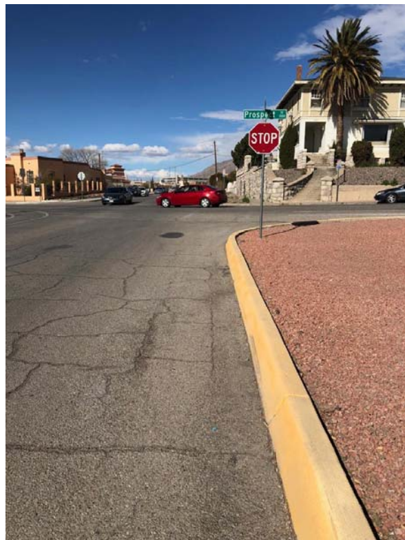
Figure E-4. Missing sidewalk and traffic control on Lawton Dr.
