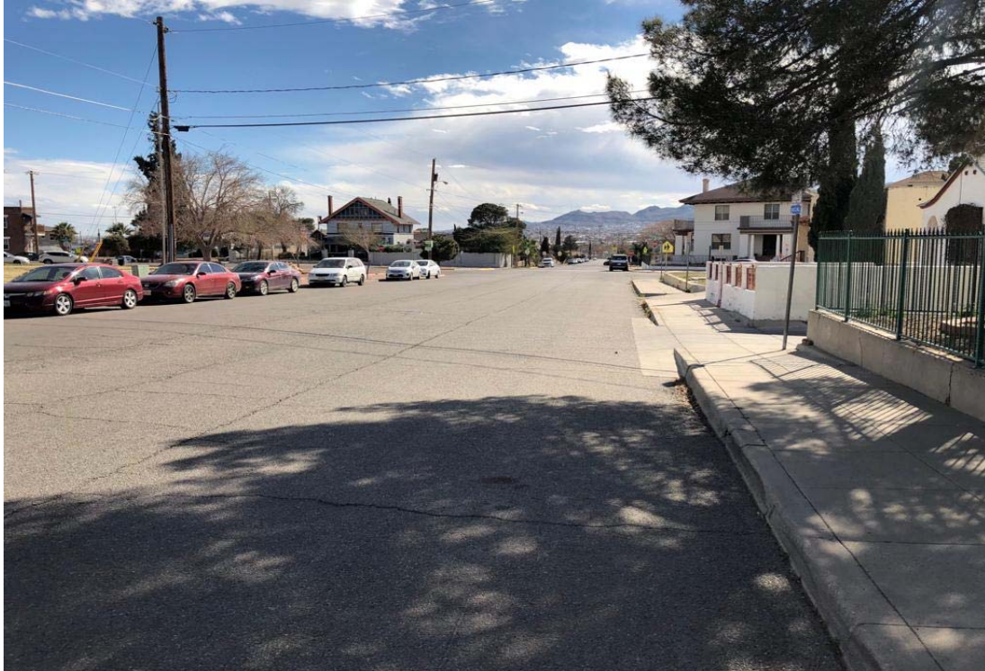
Figure C-5. Poor Illumination Rating since there is no lighting on Porfirio Diaz St.
