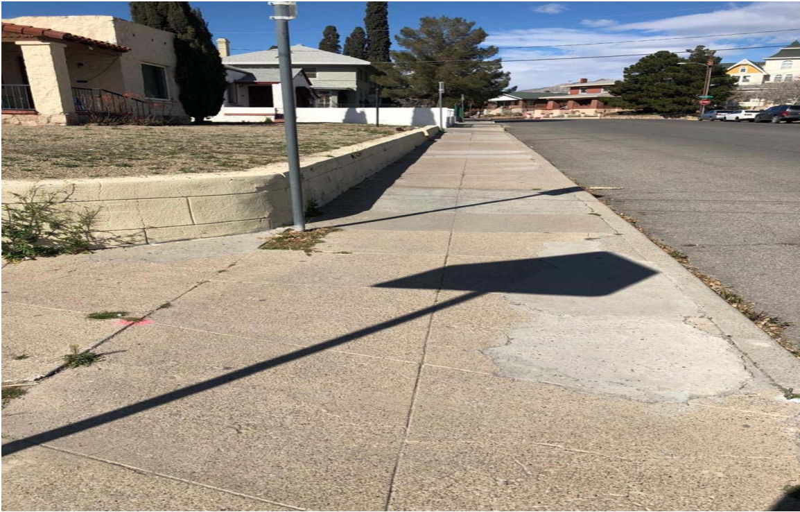
Figure C-2. Sidewalk in general good condition on Porfirio Diaz St.
