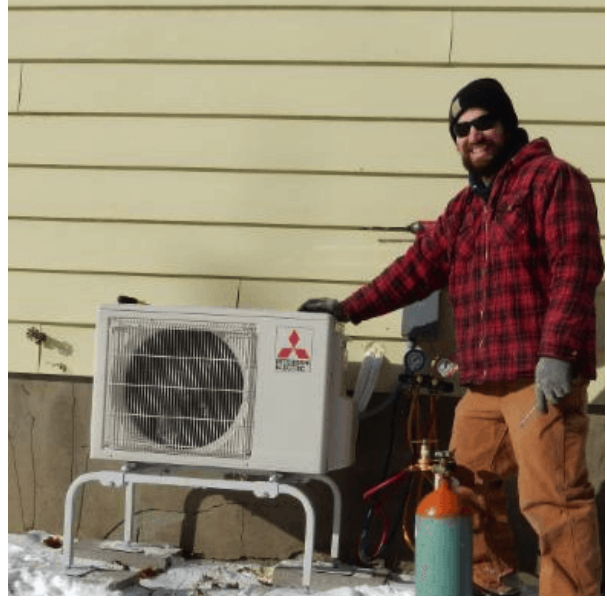
Figure 3.5: The indoor and outdoor units of a ductless mini-split heat pump. Refrigerant lines connect the units through a roughly 8 cm (in diameter) hole in the wall. Photo credit: greenbuildingadvisor.com .
