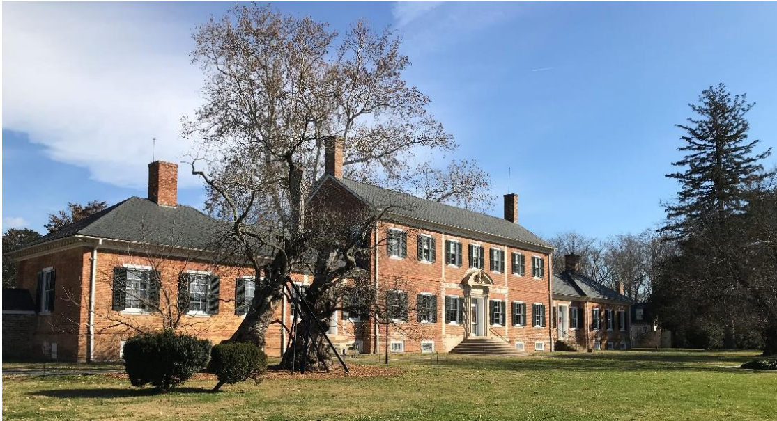
Illustration 1. A view of the west façade of Chatham Manor, which overlooks the Rappahannock River. In this view the remains of the former portico and porches remain evident. (Author's Photograph)
