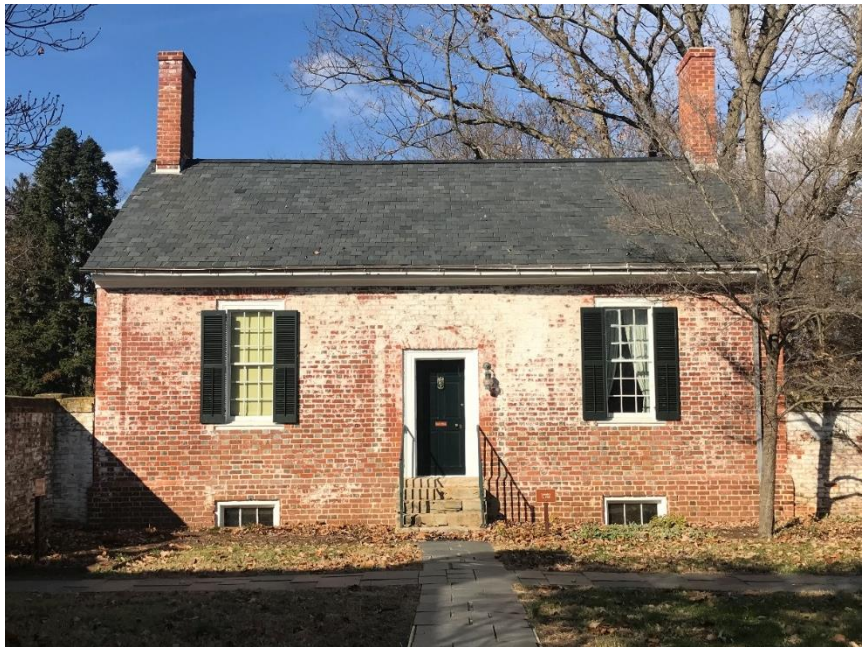
Illustration 5. This photograph shows the south façade of the laundry at Chatham Manor. The kitchen is directly opposite of the laundry and identical, with the exception of the addition of three dormers on the south façade. (Author's photograph)
