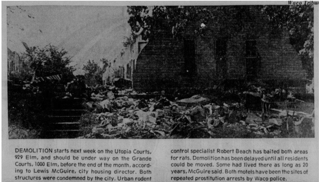
Illustration 4.4. Demolition of the Utopia Courts. The Waco Tribune-Herald .
