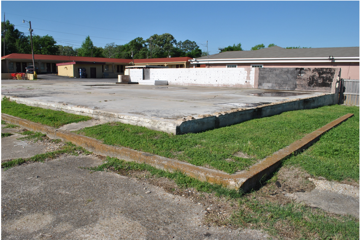
Illustration 8.18. Foundation walls at the American Inn in Tyler. Photo by Author.
