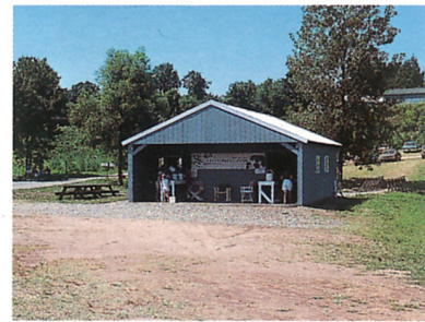
Photo 168. PYO checkout building.
