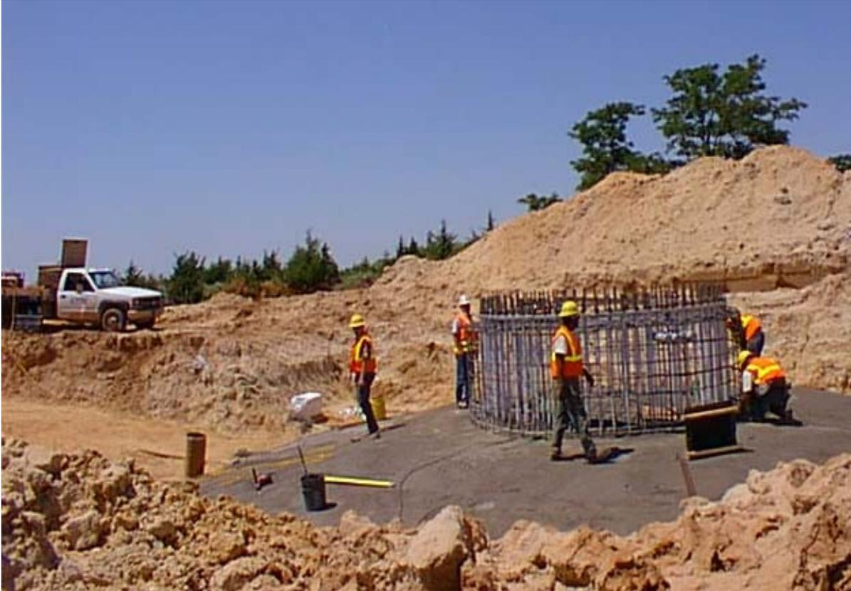
**Photo 2.** Constructing a wind turbine foundation in Woodward County, Oklahoma
