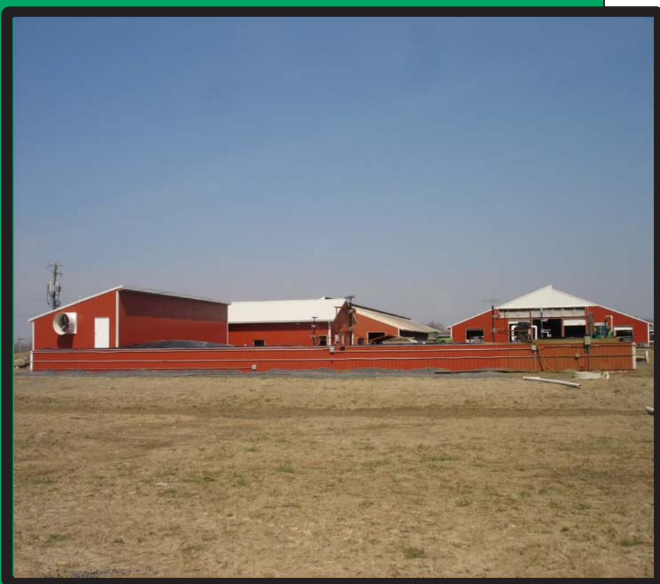
Southern perspective of digester
