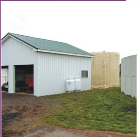
Equipment building (left); AFFD (center); long term storage (right).
