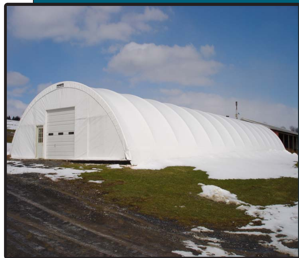
Hard top digester covered by greenhouse structure
