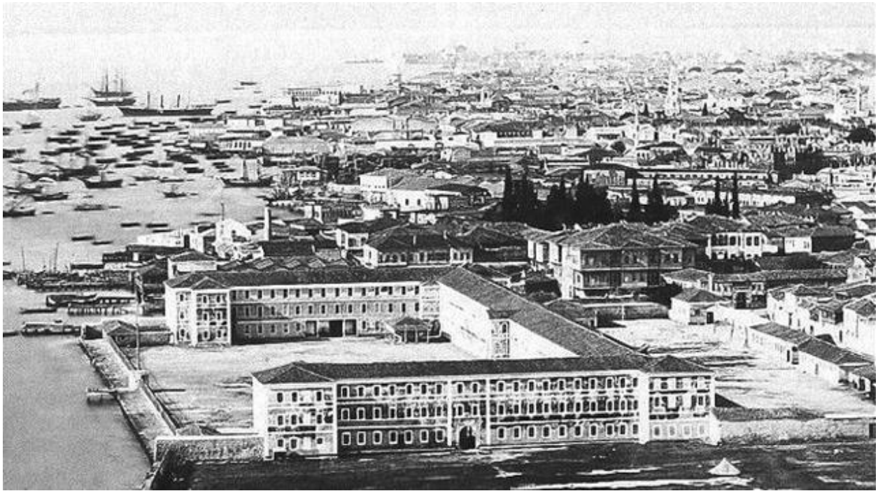
Figure 7.3 Army Barracks in Izmir, known as Kışla-i Hümayun or colloquially as Sarıkışla. Built in 1829, demolished in 1953.
