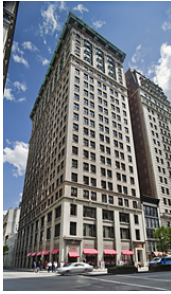
Figure 6. Site B Exterior Building
