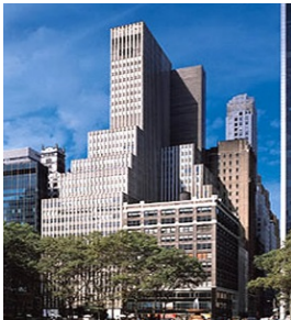
Figure 5. Site A Building Exterior
