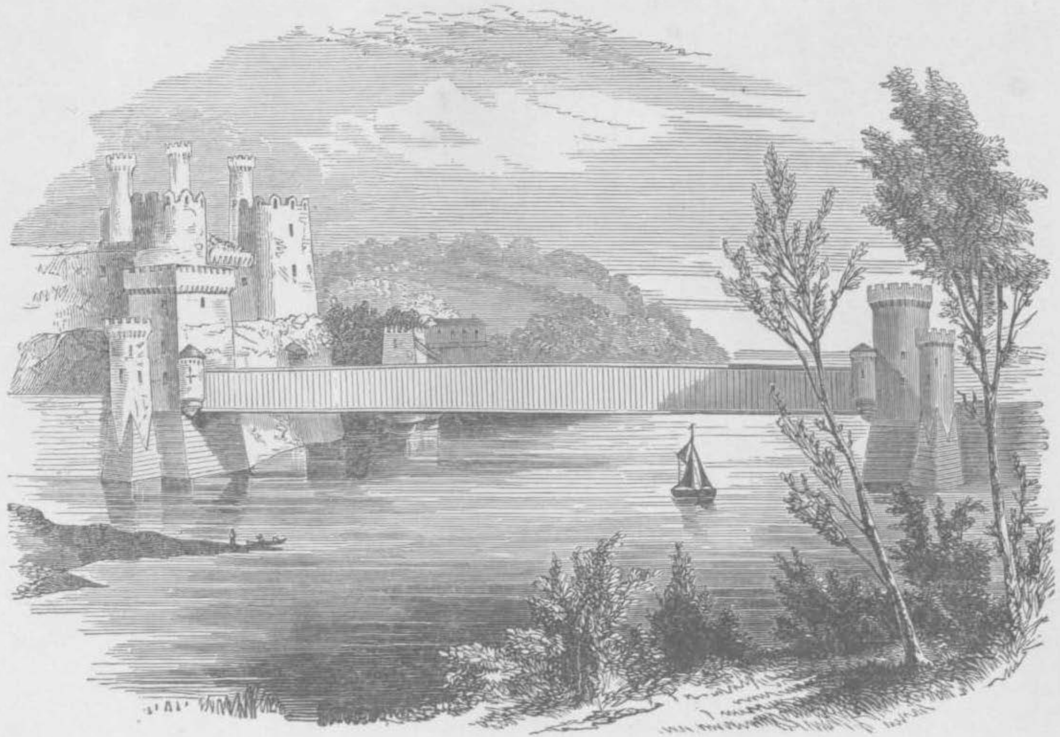
THE CONWAY TUBULAR BRIDGE.
