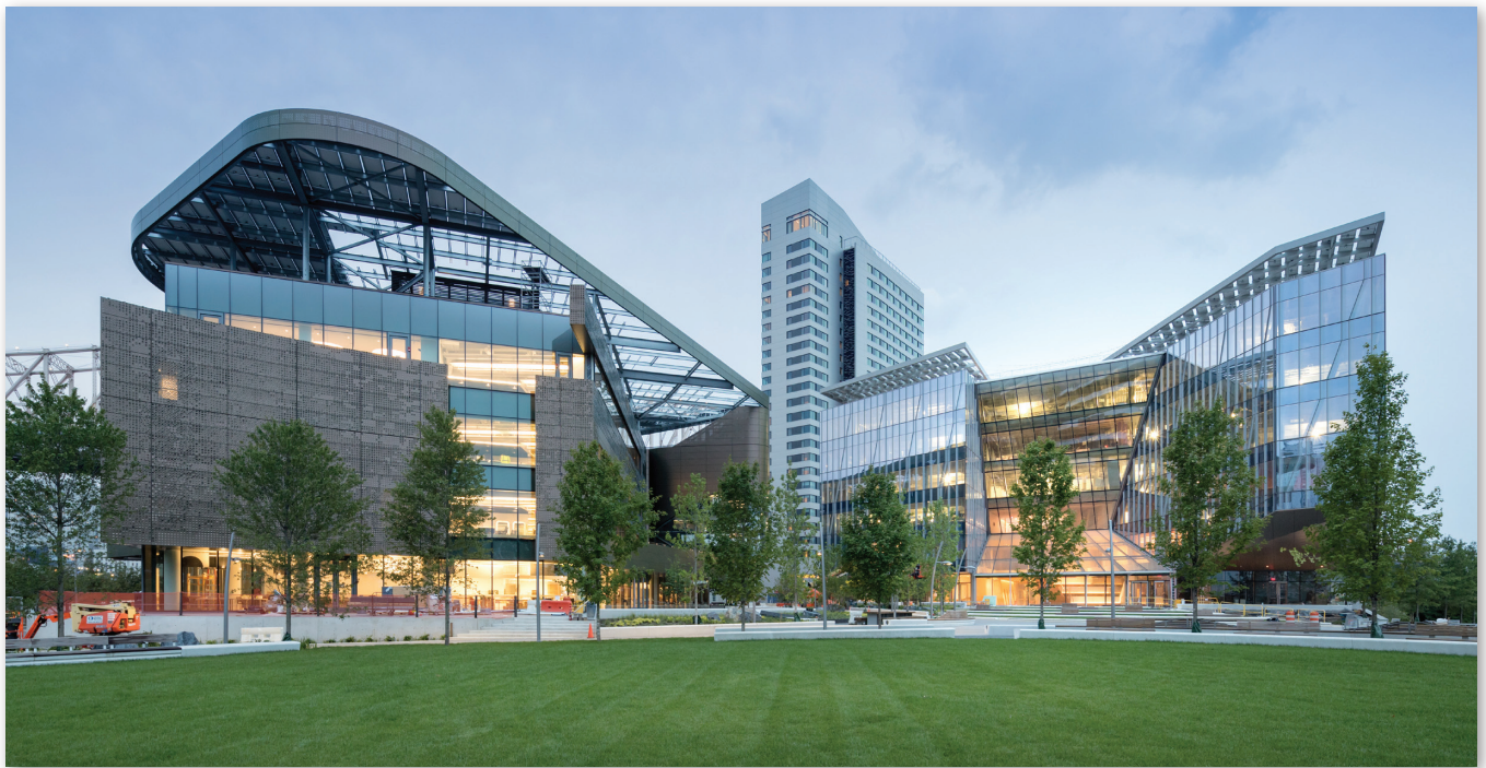
ON AN ISLAND: In September, Tech marked the opening of its first three buildings: the Bloomberg Center (at left in above photo), a residential tower called the House (at center), and an office building, the Bridge (at right). Bottom right: Students outside the Bridge. Opposite page: Funded by a $100 million gift from former New York City mayor Michael Bloomberg, the four-story Bloomberg Center is the campus's main academic building.
