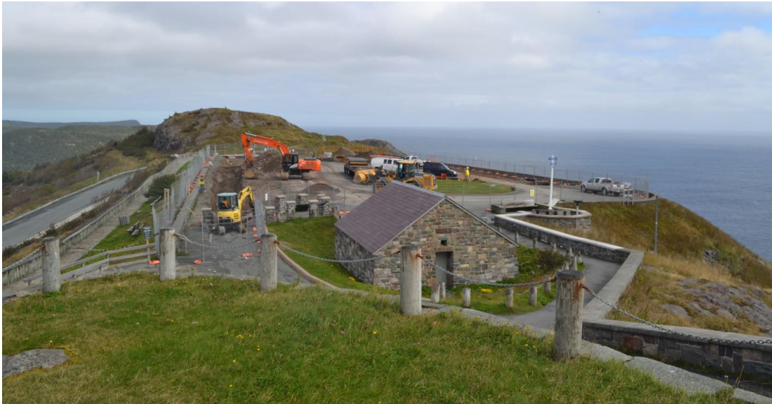
Figure 6.6. The parking lot expansion in progress, September 2016. From the author.
