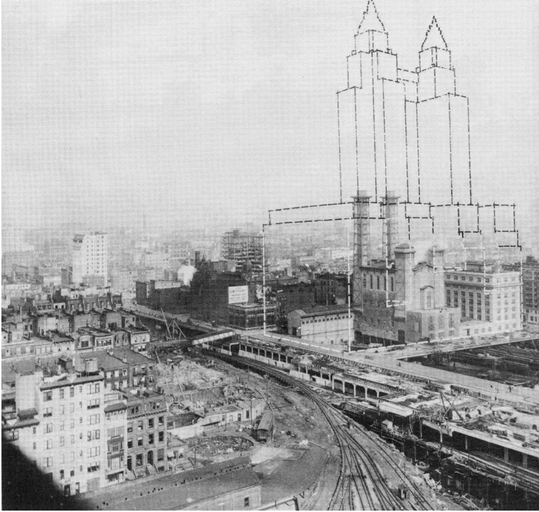
Figure 3. Grand Central Terminal, track approach during construction showing outline of future Waldorf-Astoria Hotel, 1911. (Condit, Port of New York , 2:88)
