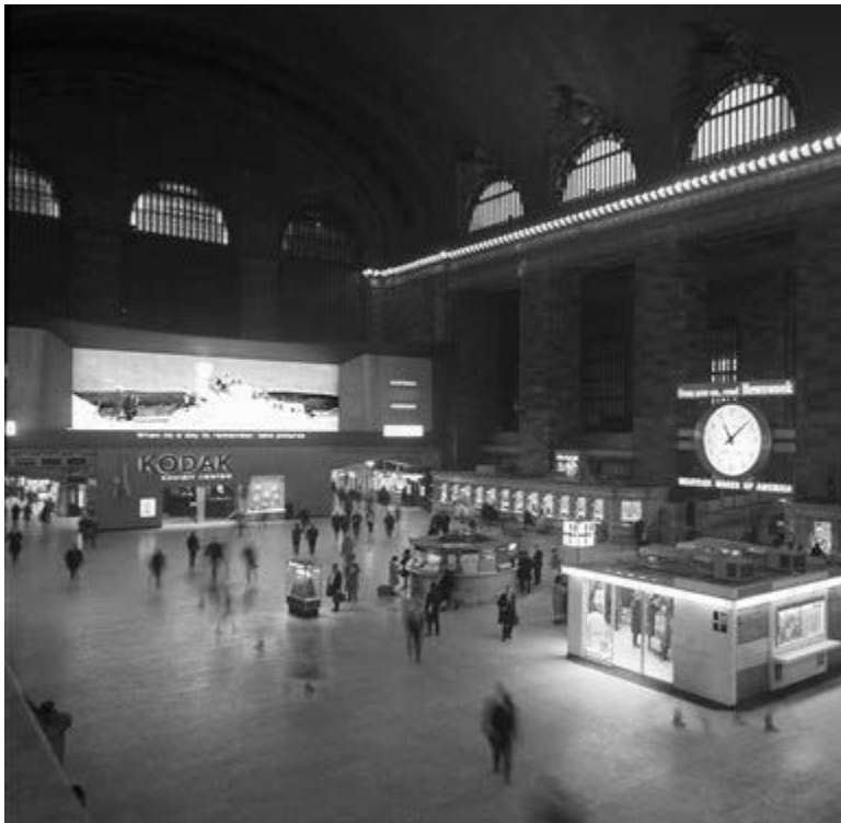
Figure 10. Grand Central Terminal, concourse with advertisements for Kodak, Westclox, and Merrill Lynch, 1968. (AP Photo)
