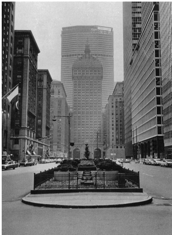
Figure 34. Above left : Cover of New York magazine illustrating demolition of the Pan Am Building, 1987.
