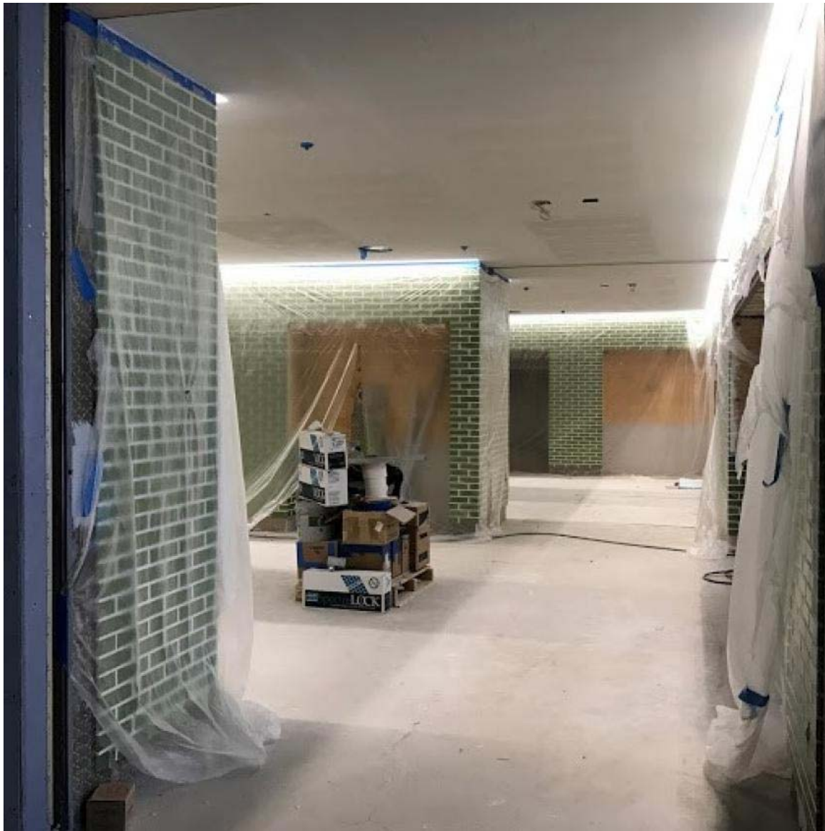
Tile work in new cafeteria area
