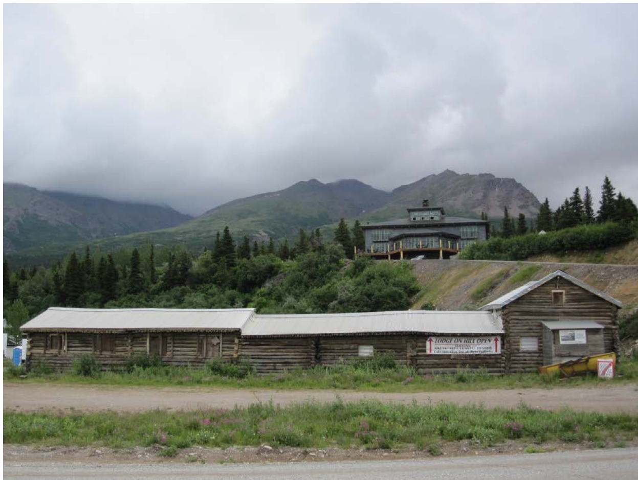
Figure 43. Historic Rapids Roadhouse with the new Rapids Roadhouse positioned on the hill above. Photo by Casey Woster.
