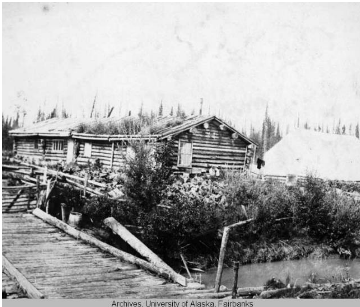
Figure 72. Pile Driver Roadhouse, undated. Edward R. McFarland Photographs, University of Alaska Fairbanks.
