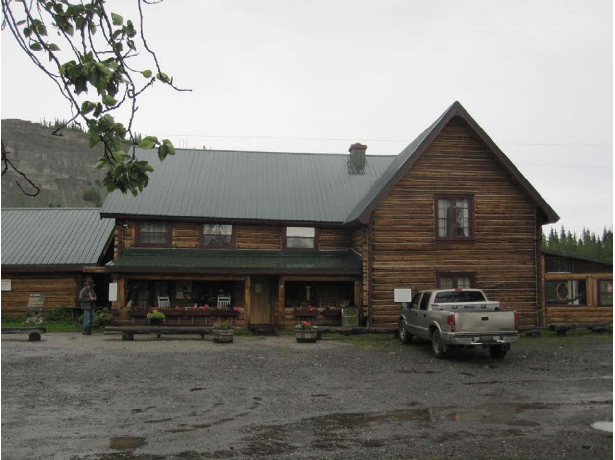
Figure 31. 1929 roadhouse building at Gakona. Photo by Casey Woster.
