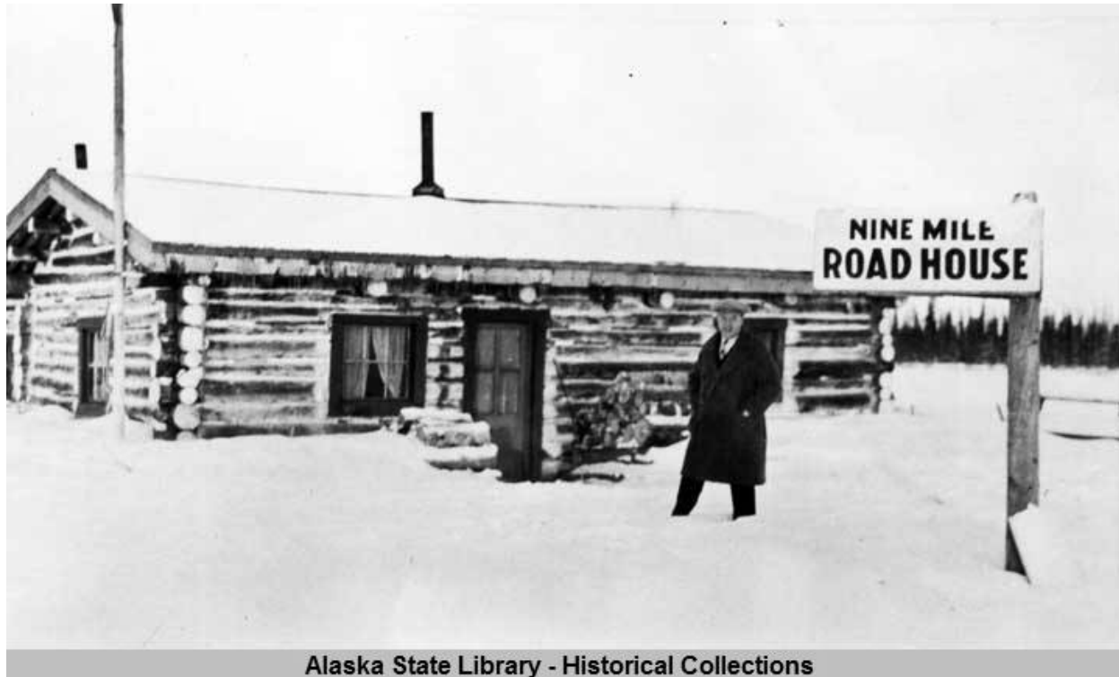
Figure 75. Ninemile Roadhouse, undated. Ira and Walter Wood Photograph collection, ca. 1911-1929, Alaska State Library, Historical Collections.
