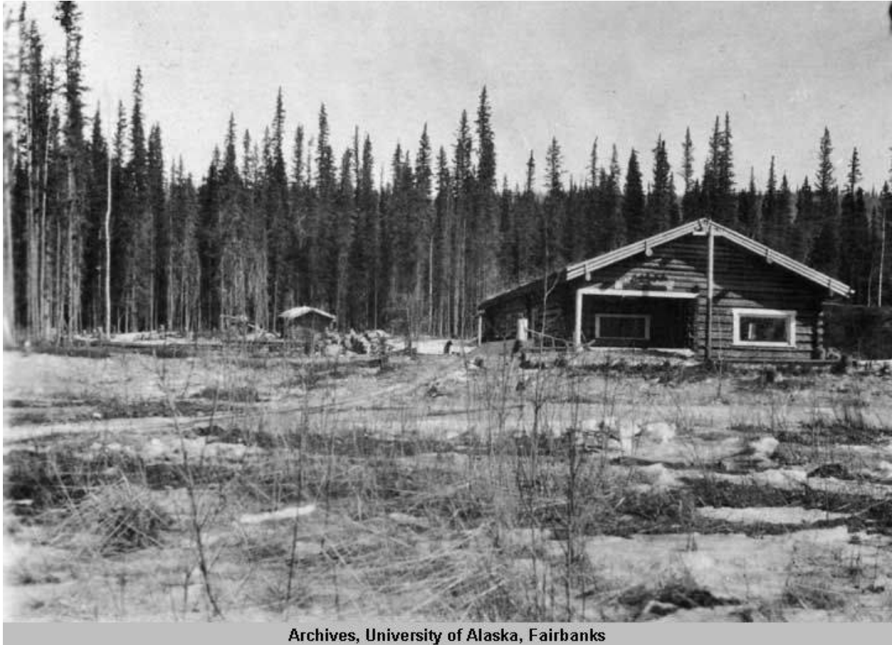
Figure 69. Silver Fox Roadhouse, undated photograph. Drane Family Collection, University of Alaska Fairbanks.
