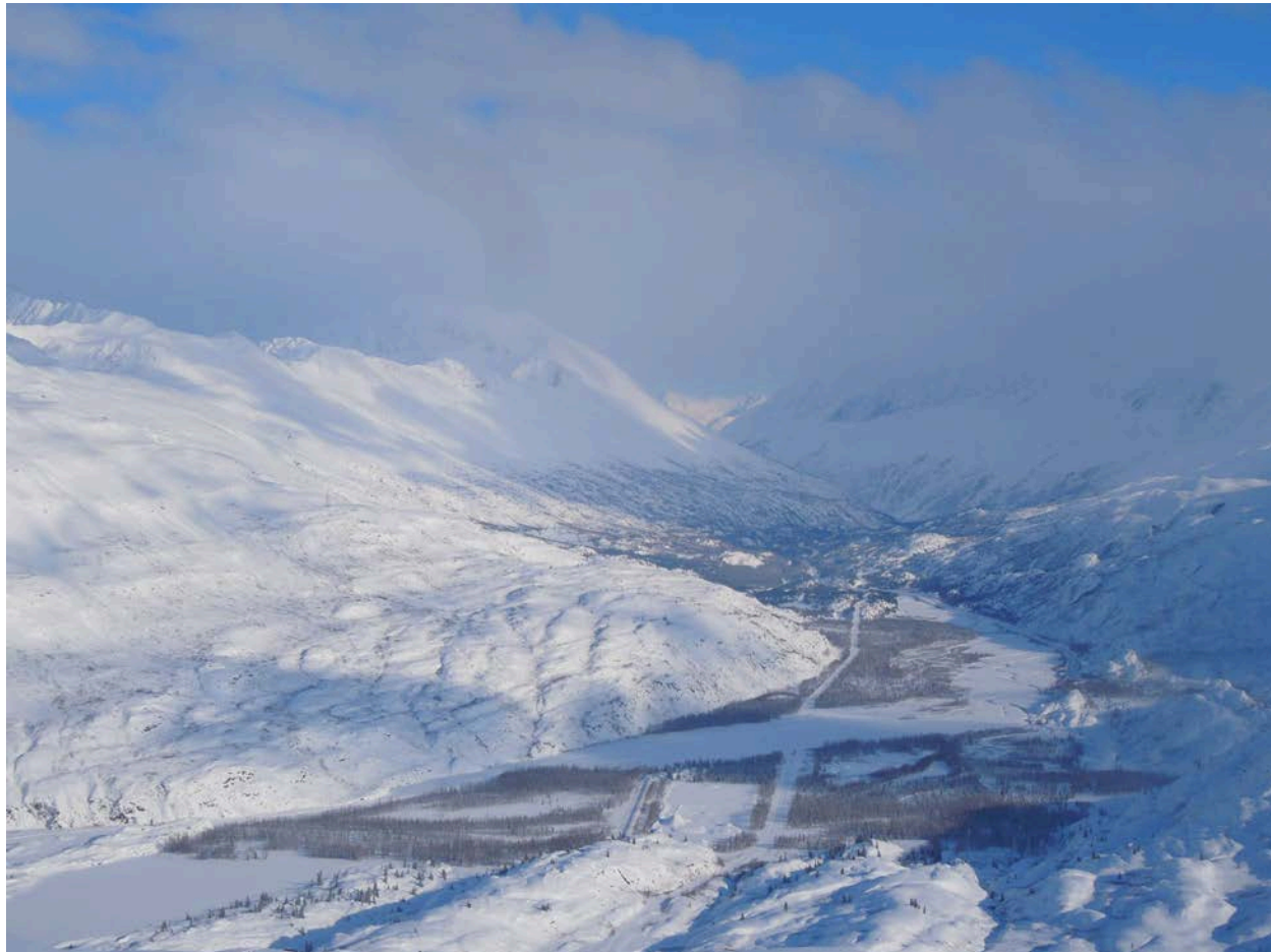
Figure 12. Thompson Pass from the surrounding mountain ridges, showing the cleared space for the Trans Alaska Pipeline. Photo courtesy of Scott Woster.
