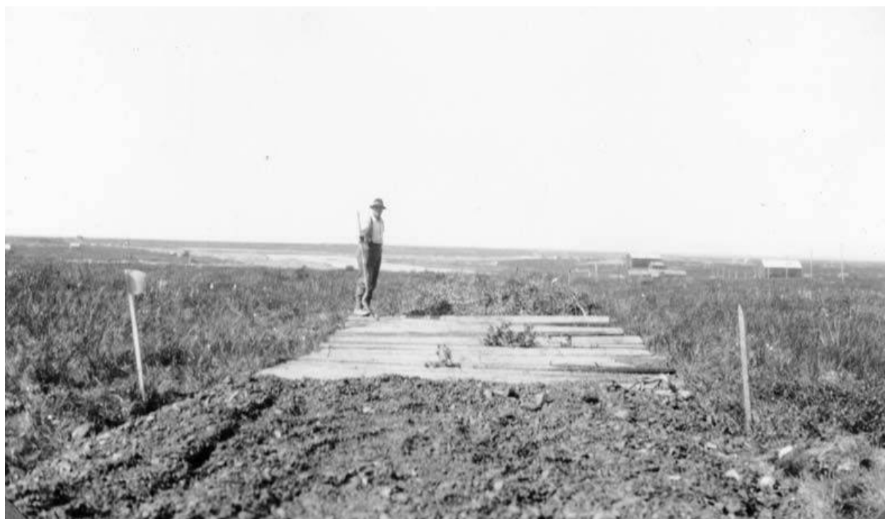
Figure 17. Corduroy road construction, ca. 1930s. Walter Hodge Papers, University of Alaska Fairbanks Archives.
