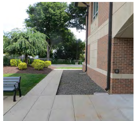
A two-foot wide vegetation free zone around buildings can reduce moisture problems. Photo: M. Frye
