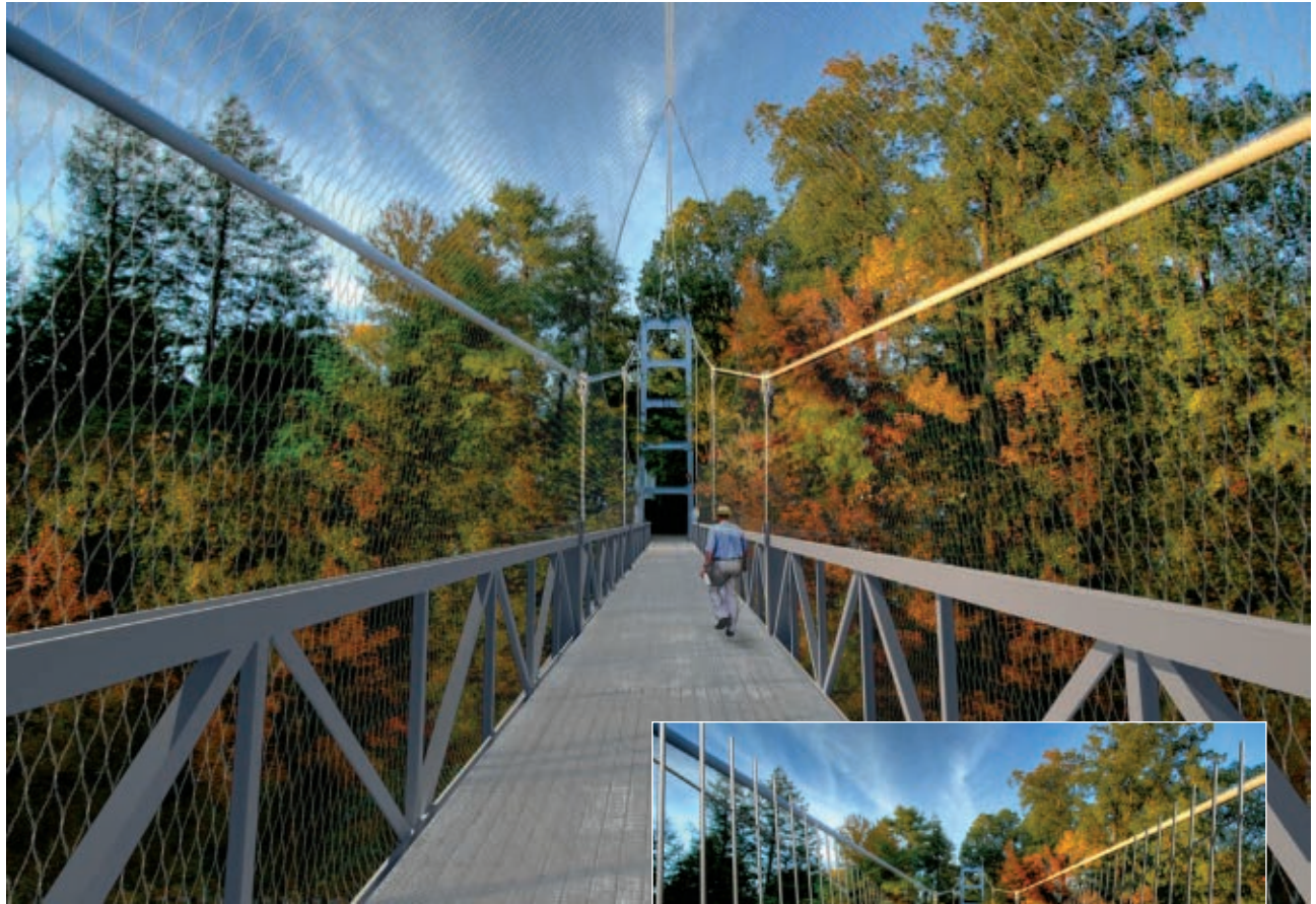
Means restriction: Potential methods for preventing suicides on the Suspension Bridge include fine wire mesh fencing (above) and vertical barriers (right).
