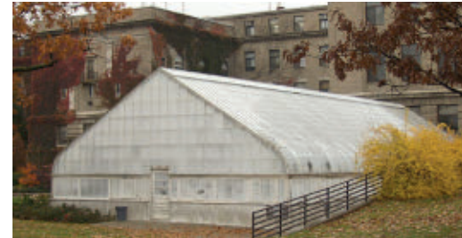
Growing pains: The Bailey Hortorium is facing the wrecking ball. Left: A Thirties-era ad for architects Lord & Burnham.
