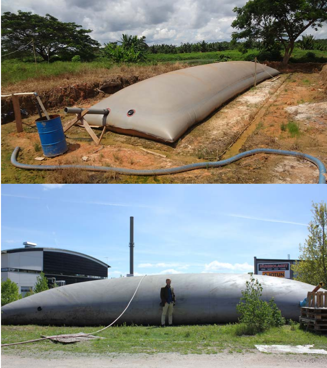
Figure 9: Multiple views of the bladder-like material that is used to produce a FOV Biogas anaerobic digester (Source: FOV Biogas)
