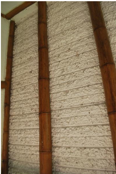
Figure 10: Example of walls made of Guadua, Metallic mesh and Mortar 85 .
