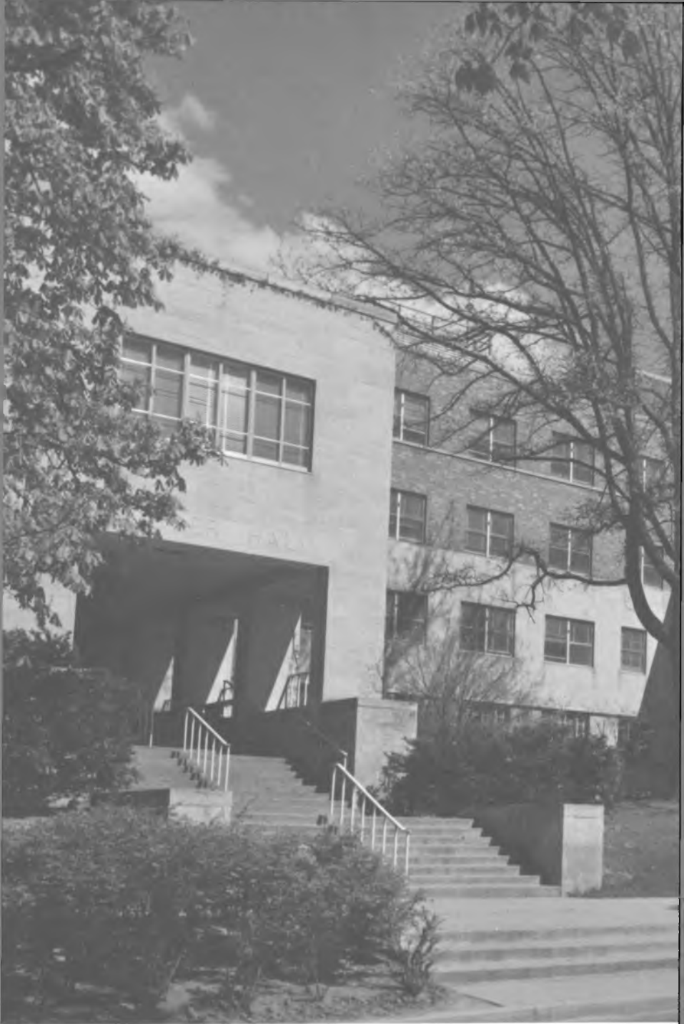
Statler Hall, home of the School of Hotel Administration, is constructed in three sections. The building's central section, shown above, is entirely given over to classrooms, laboratories, and offices. The School's library, student lounge, and
