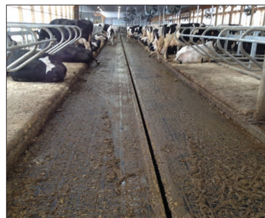
GEA tube scraper system
