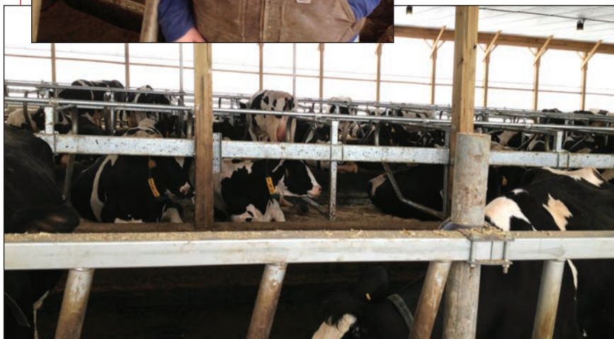
Above: Jen Dubina, herd manager. Below: GEA FT patented single beam freestall mounting system.
