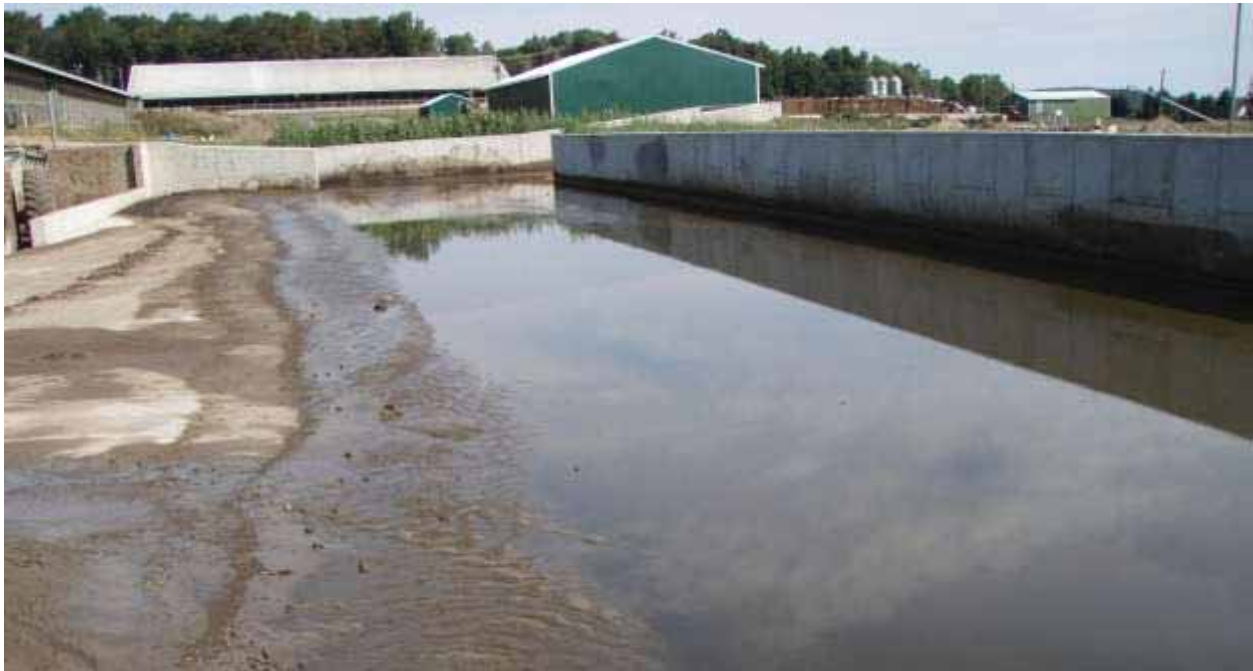
Photo 3. Completed Sand Lane
