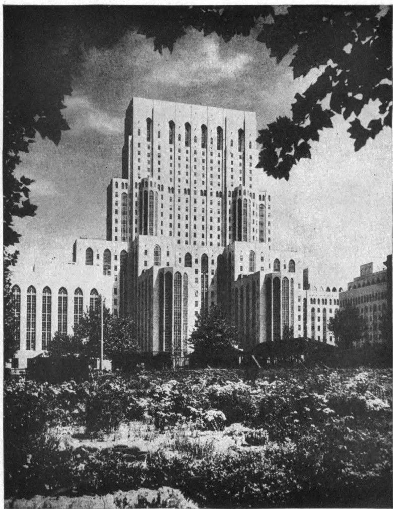
THE NEW YORK HOSPITAL, SOUTH VIEW
