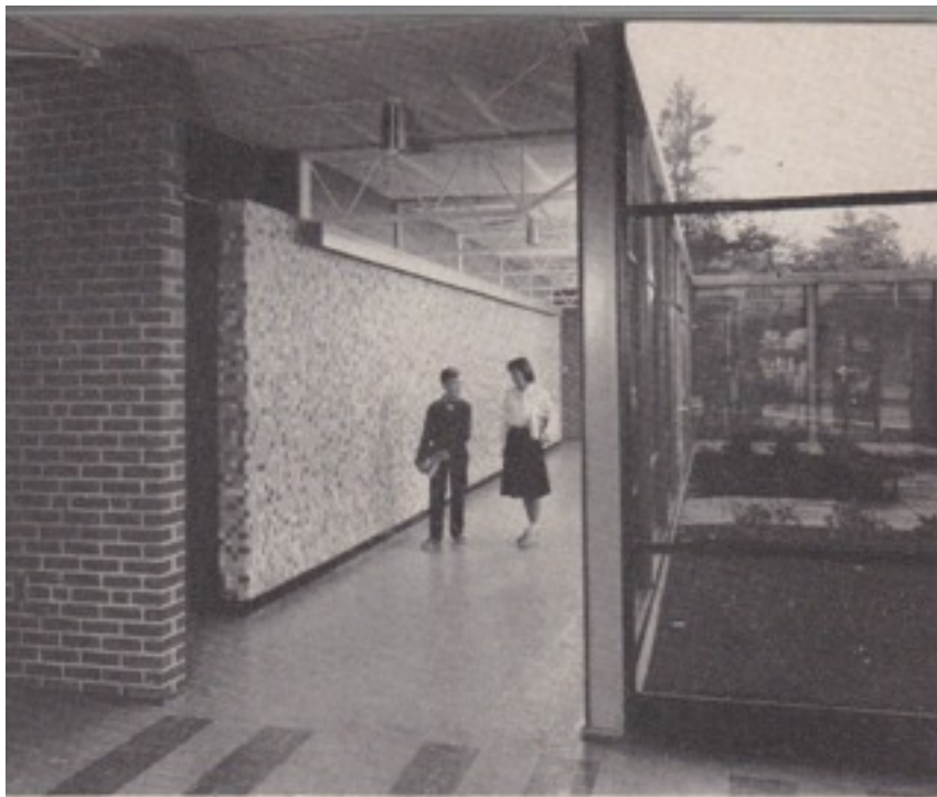
Figure 6.10. South Elementary School [1961] Hugh Stubbins & Associates, architect; Andover, MA in "Courts Enhance Environment of Low Cost School," Architectural Record 130, no. 1 (Jul. 1961): 167; PhotoCrd: Joseph W. Molitor.
