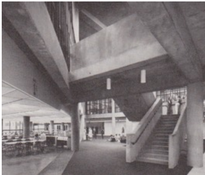
Figure 5.12. Barnstable Middle School [1979] Caudill, Rowlett, Scott, architects; Hyannis, MA in “Schools,” Architectural Record 165, no. 7 (Jun. 1979): 133; PhotoCrd.: Nick Wheeler.
