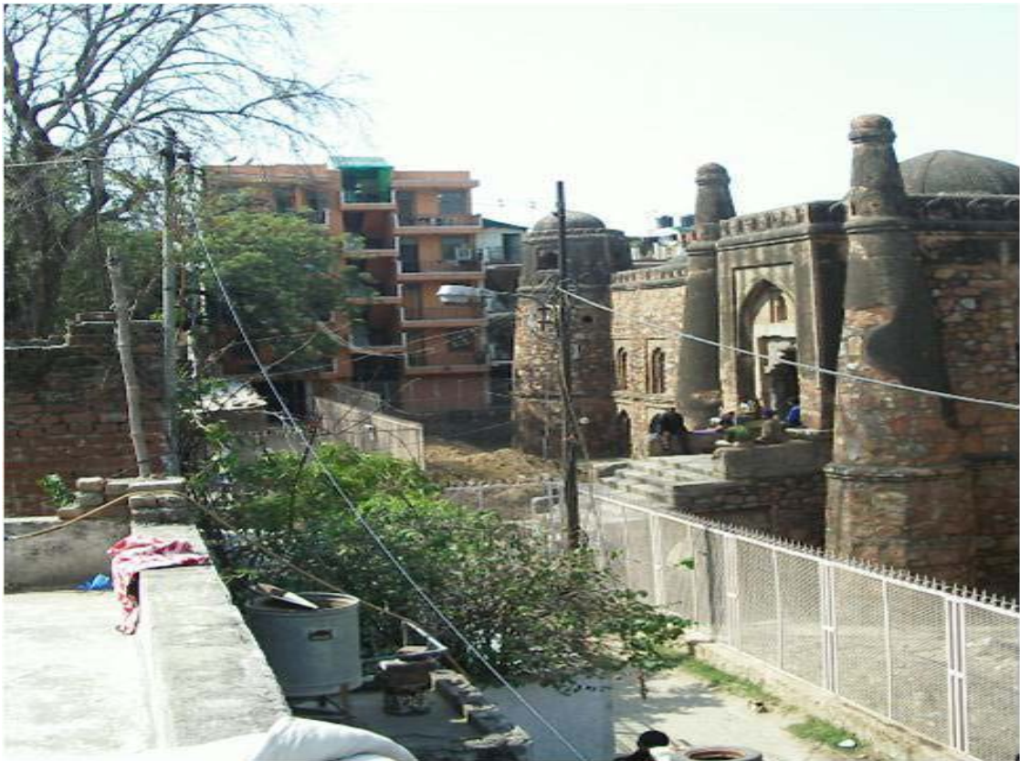
Figure 3.03: The South face of the Khirki Mosque around which the village now exists.
