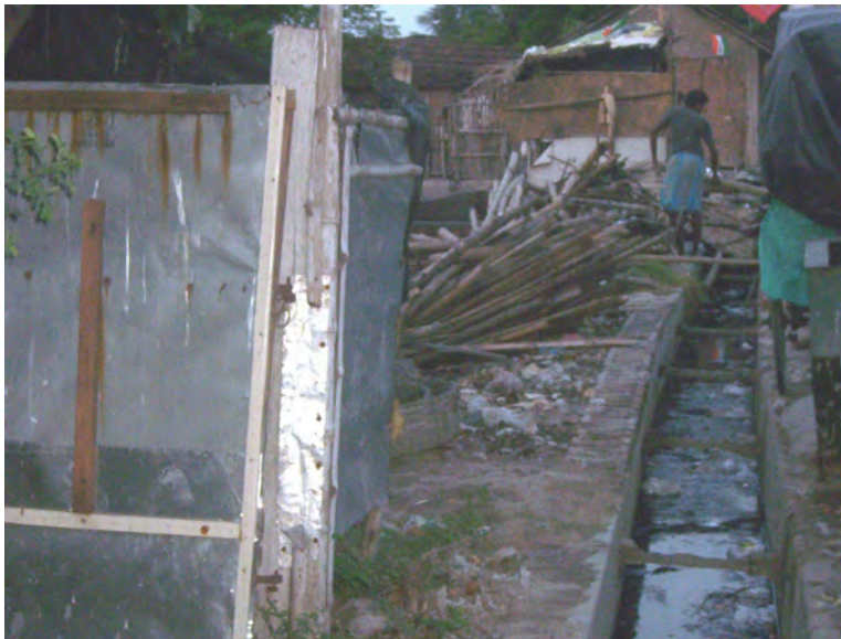
Figure 5.5: Open drains - Duttabad
