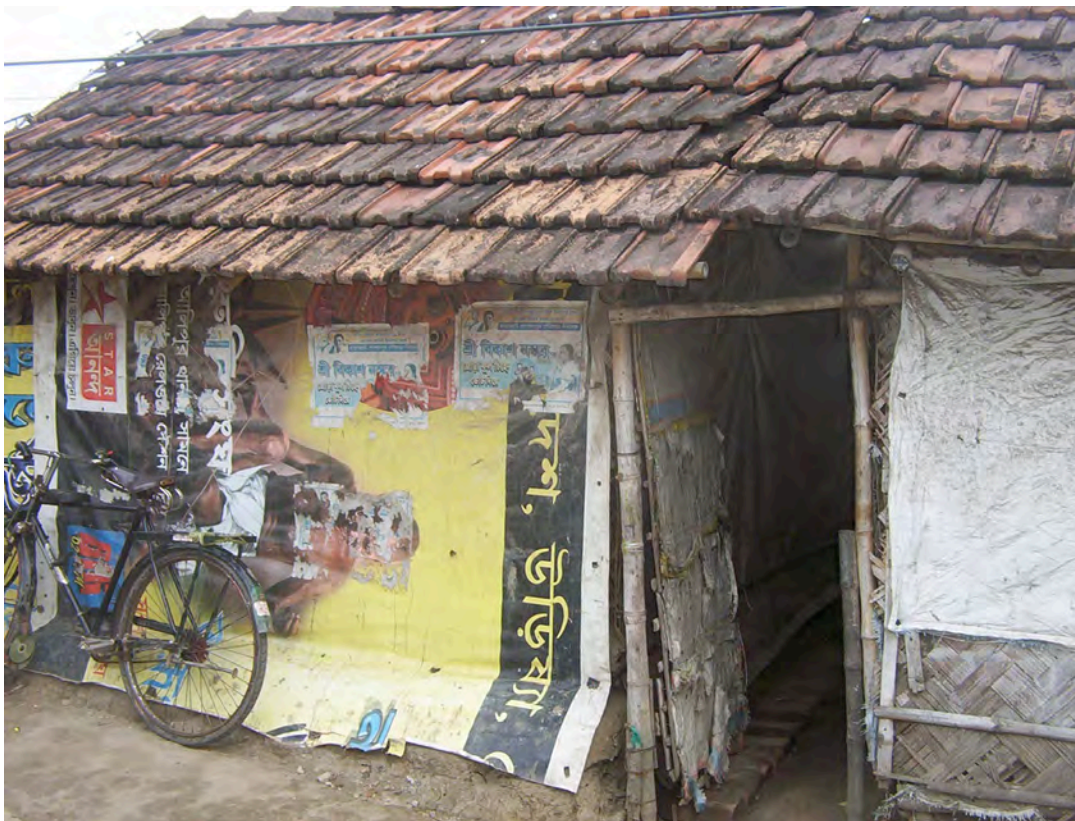
Figure 5.2 – Semi-pucca housing structure in the Nayapatti settlement
