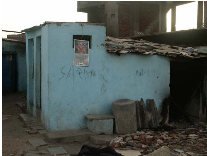
Figure 61. Incorporation of the Muslim into the Hindu. Part of a destroyed Muslim residence at Naroda Patia, a few days after the massacre. The coal scribbles say, “ Jai Shri Ram ” (Hail to God Ram) and the image of Goddess Ambaji has been attached to the wall.
