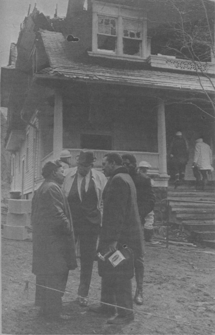
ON SITE INVESTIGATION — Investigation into the fire at 320 Wait Avenue, burned out home of the Africana Studies and Research Center, continued over the weekend. On Saturday, Chester Whiteside, an arson investigator from the Syracuse Police Department, joined the investigation team. Whiteside, with lamp and briefcase, talks with J. Congress Mbata, Africana Studies associate professor, far left, while Ithaca Police Chief Herbert L. VanOstrand, in light coat, and James Cunningham, Africana Center writer-in-residence, look on.
