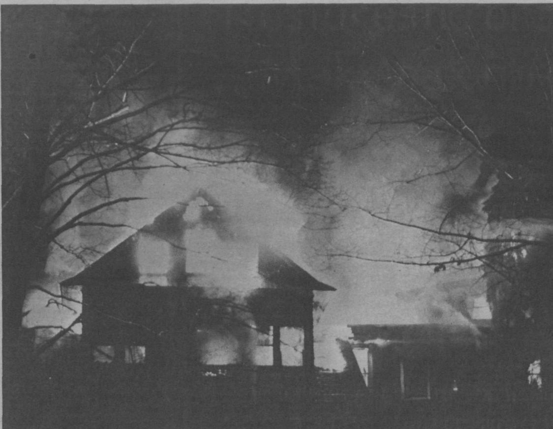
FLAMES AT 320 WAIT — Flames leap from upper floors of building at 320 Wait Avenue housing Africana Studies and Research Center which was swept by fire early Wednesday morning.
