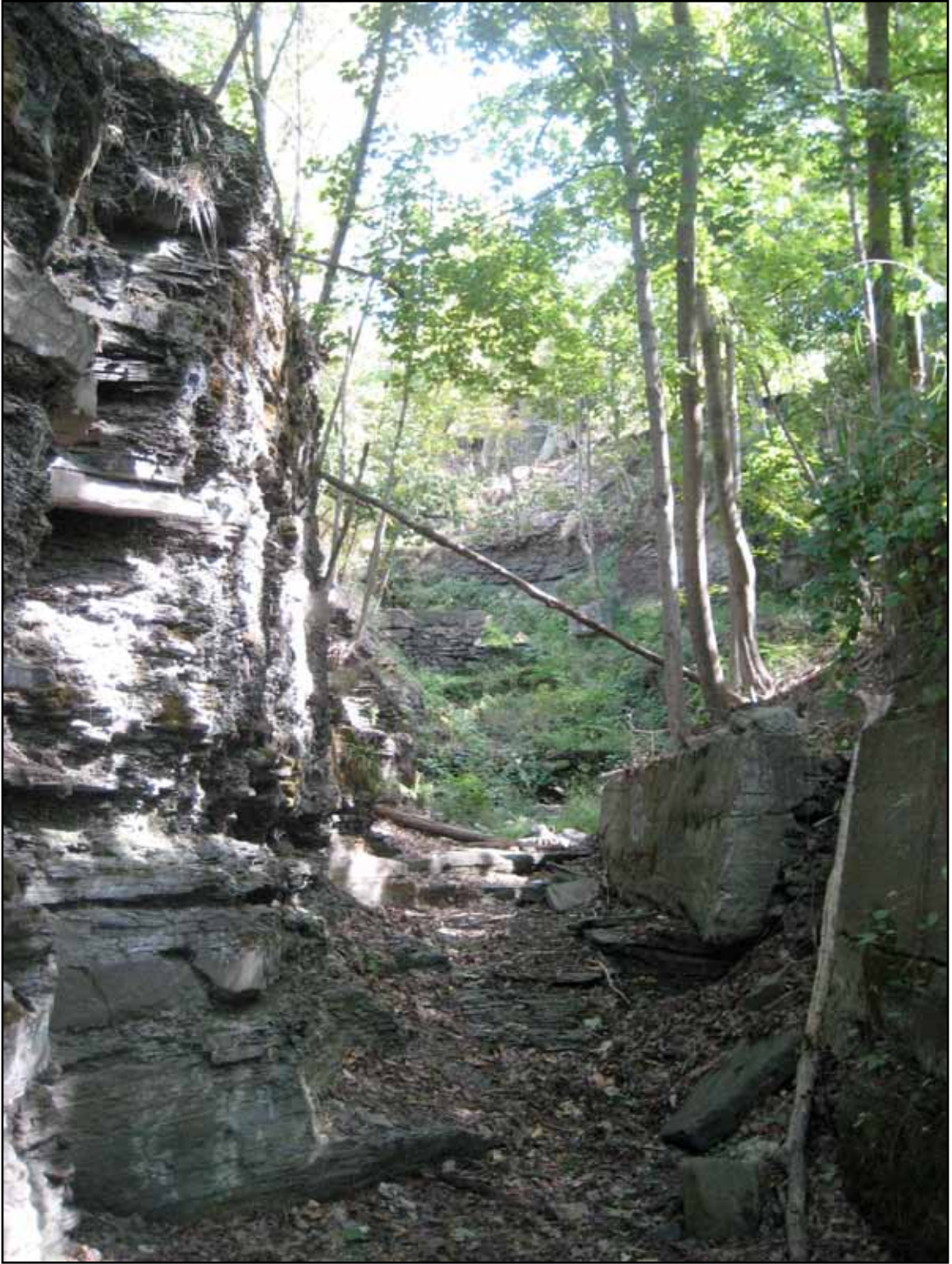
Fig. 113. Looking southeast through the raceway at the point where it makes a forty-five degree turn. (Photograph by author).
