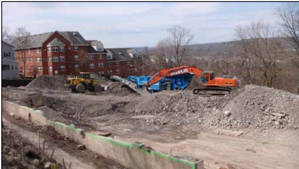
Fig. 63. Main factory debris removal. (Photograph by Leigh McGonagle, April 18, 2009).
