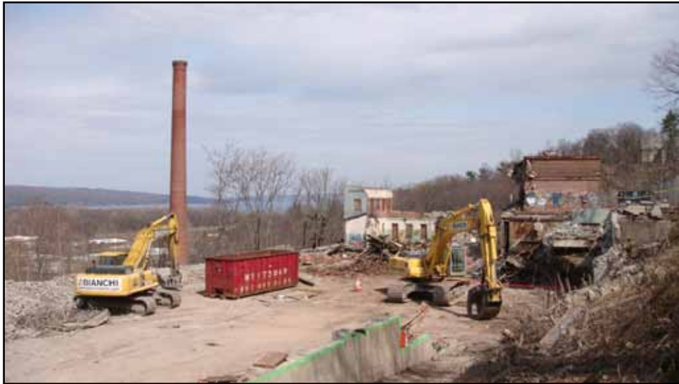
Fig. 62. Demolition of main factory building. (Photograph by Leigh McGonagle, April 18, 2009).
