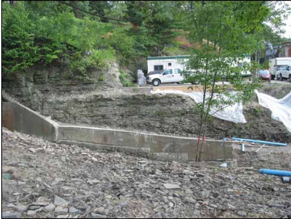
Fig. 48. EPA cleanup of upper raceway, stripped to bedrock. (Photograph by Liska Clemence, 2003, courtesy of Kathryn Gleason).
