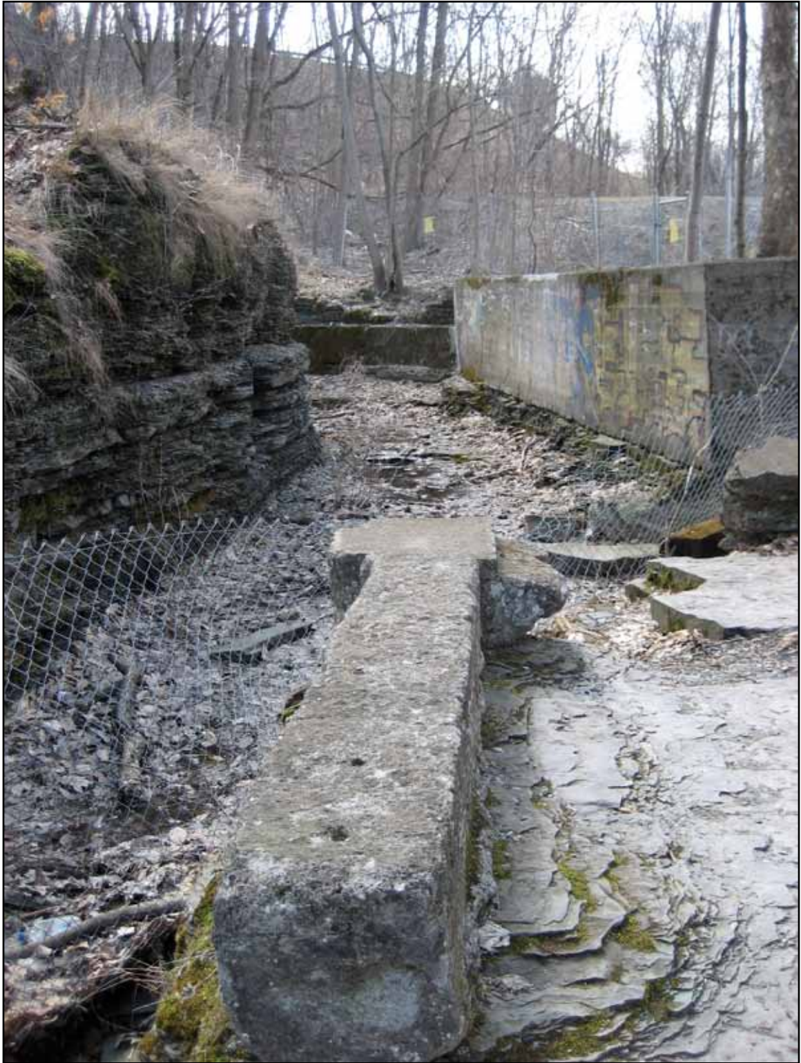
Fig. 114. Looking south from the top of the flume to the flour mill. The western side of the raceway is formed by a concrete retaining wall, while the eastern side is cut from the rock at the base of the Island (Photograph by author).
