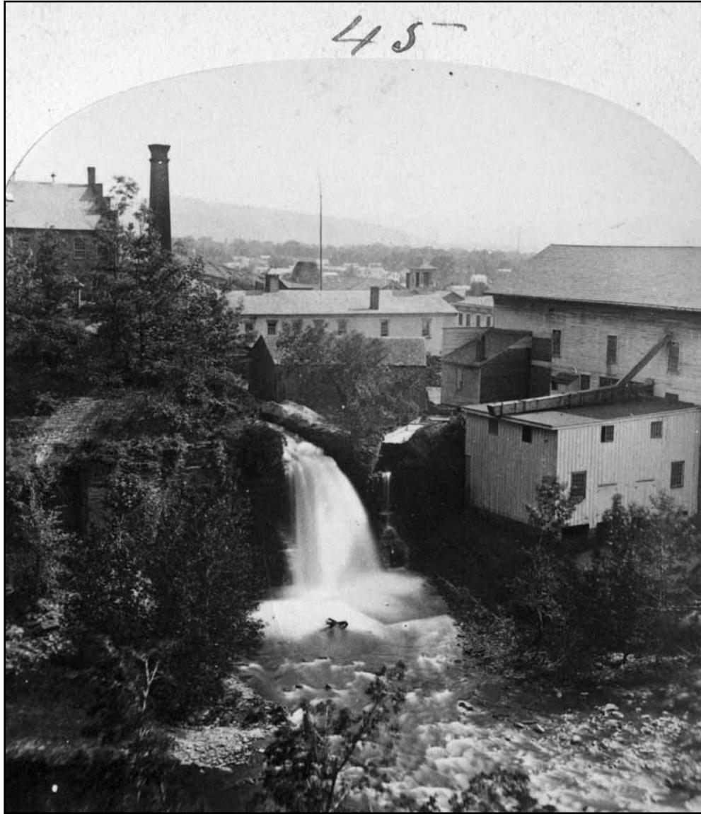
Fig. 16. View looking south from the northern gorge ridge of the Fall Creek flour mill and end of raceway. (K5.75_45 : Dewitt Final)
