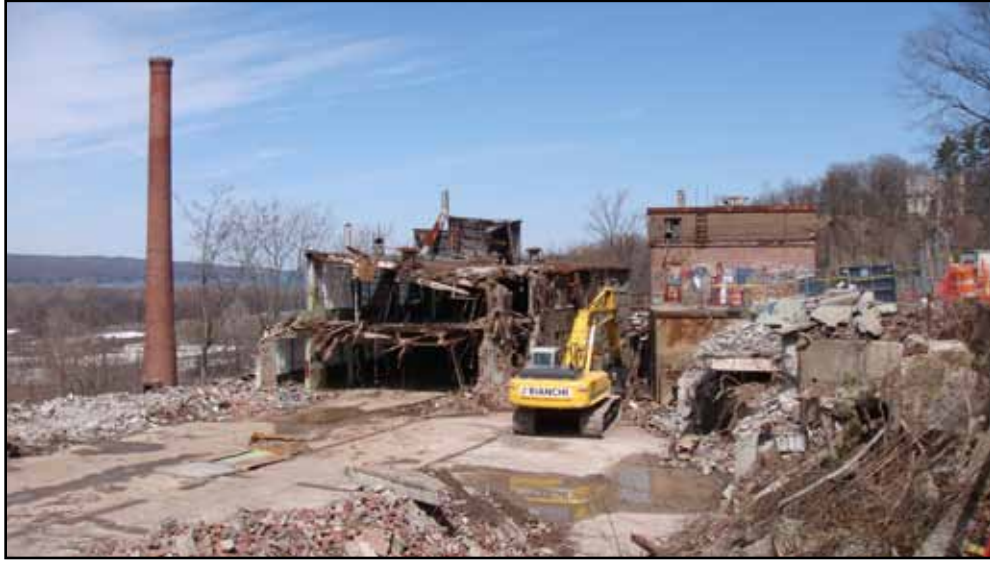
Fig. 60. Demolition of main factory building. (Photograph by Leigh McGonagle, March 27, 2009).
