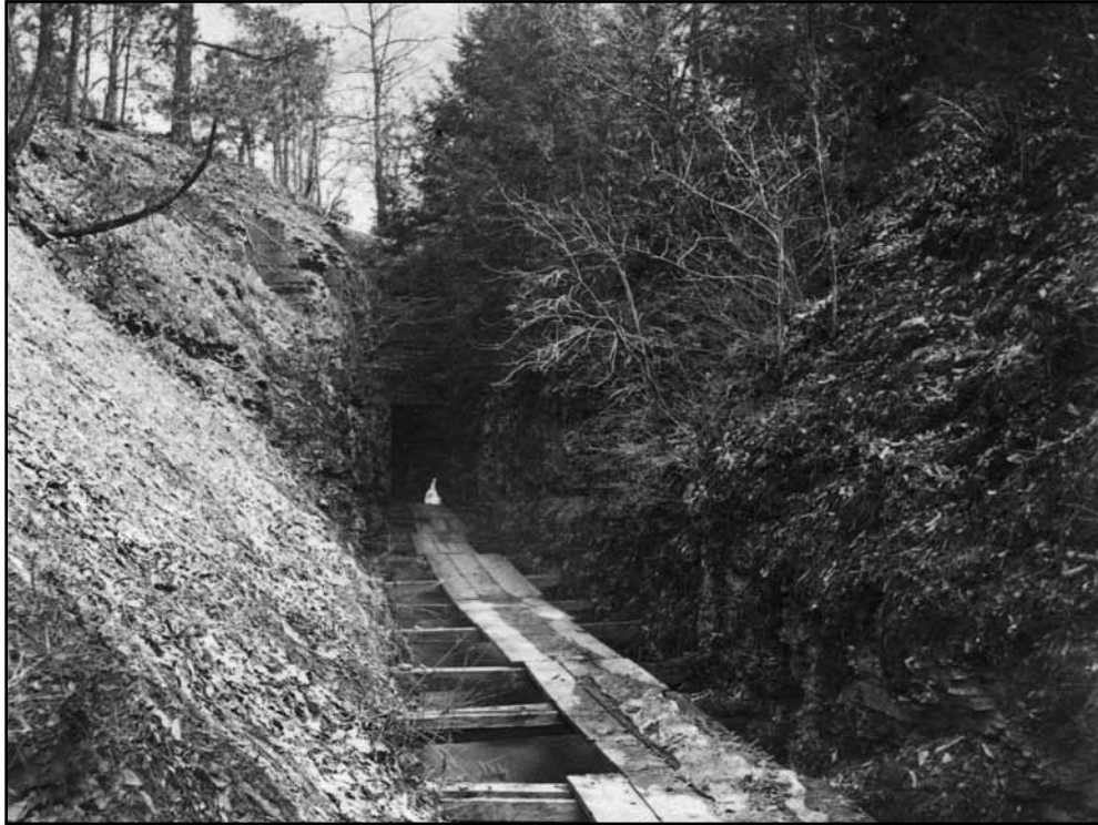
Fig. 17. View east along wooden flume towards tunnel. (R20.18 : Dewitt_Final)
