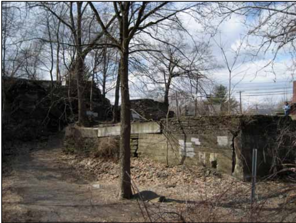
Fig. 87. Foundation of the flour mill from the creek. (Photograph by author).
