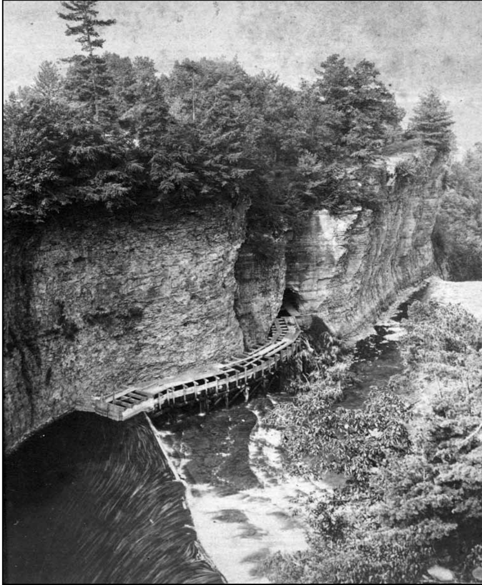
Fig. 23. Original dam and wooden flume carrying water through tunnel. (Looking_down_fr_Chimney_Rocks : Historical files)
