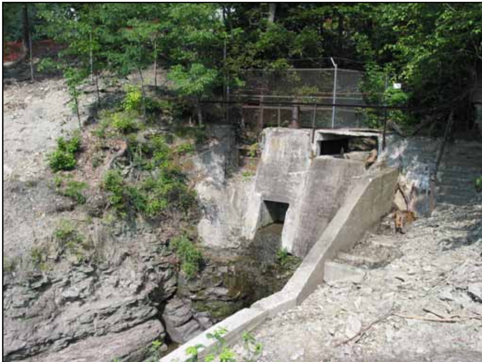
Fig. 58. Bulkhead post-cleanup. (Photograph by Liska Clemence, 2003, courtesy of Kathryn Gleason).
