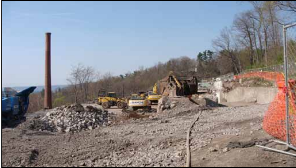
Fig. 64. Demolition of main factory building. (Photograph by Leigh McGonagle, April 26, 2009).
