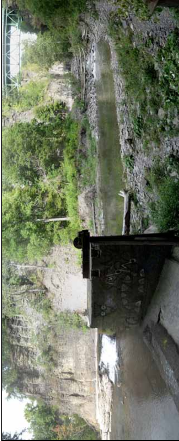
Fig. 97. View from the head of the tunnel of the dam and the lifting mechanism that allowed water to pass through. At far right are the remains of the wooden chute that carried water from the original dam to the tunnel. (Photograph by author).
