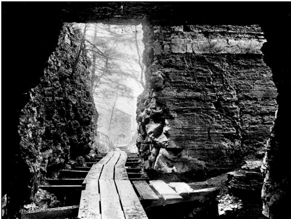
Fig. 18. View from western tunnel mouth. (Tunnel downstream : Historical_Files)
