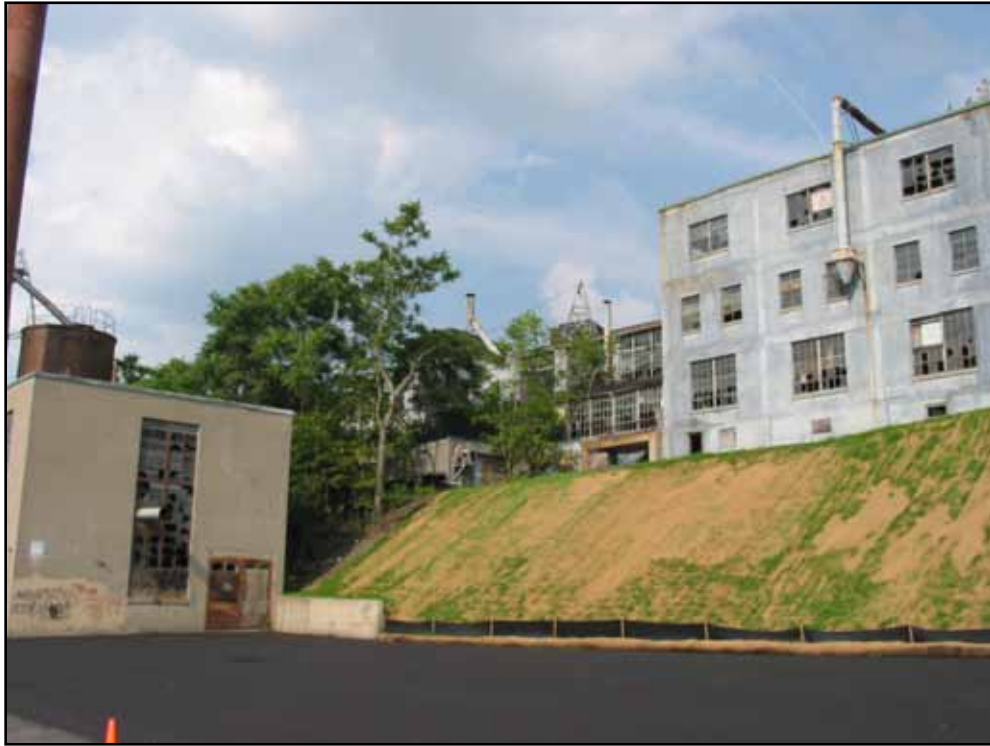
Fig. 46. Revegetation of slope below gun factory. (Photograph by Liska Clemence, 2003, courtesy of Kathryn Gleason).
