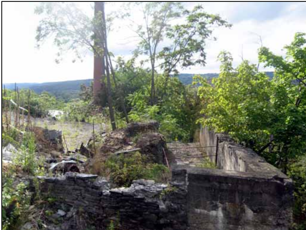
Fig. 90. Foundation of the original gun factory building, inherited from the site's predecessor, the Ithaca Manufacturing Works. (Photographed by author).
