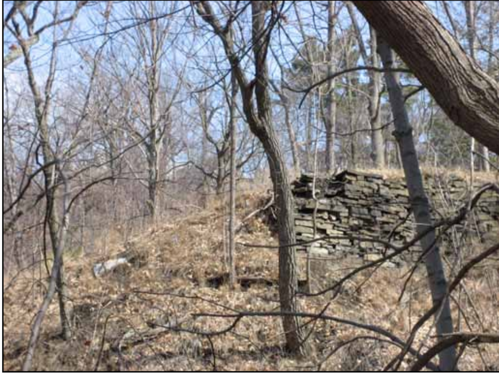
Fig. 89. Stone foundation of the bridge crossing the lower raceway to the foundry on the Island. (Photograph by author).
