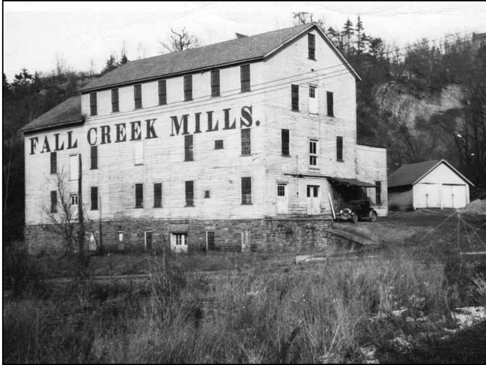
Fig. 14. View facing northeast of the Fall Creek flourmill (R20.137 : Dewitt_Final)
