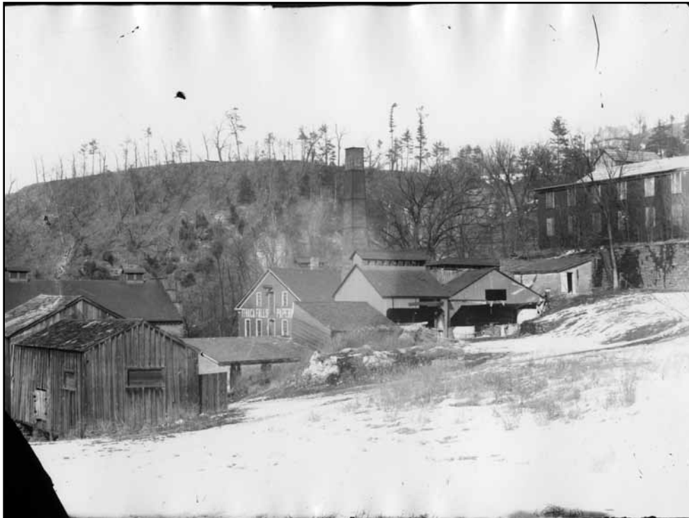
Fig. 15. View looking north from Lake Street towards the Ithaca Falls Paper Mill. (R20.101 : Dewitt_Final)
