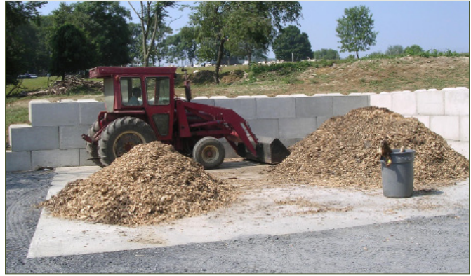
Bin made from concrete block highway dividers.
