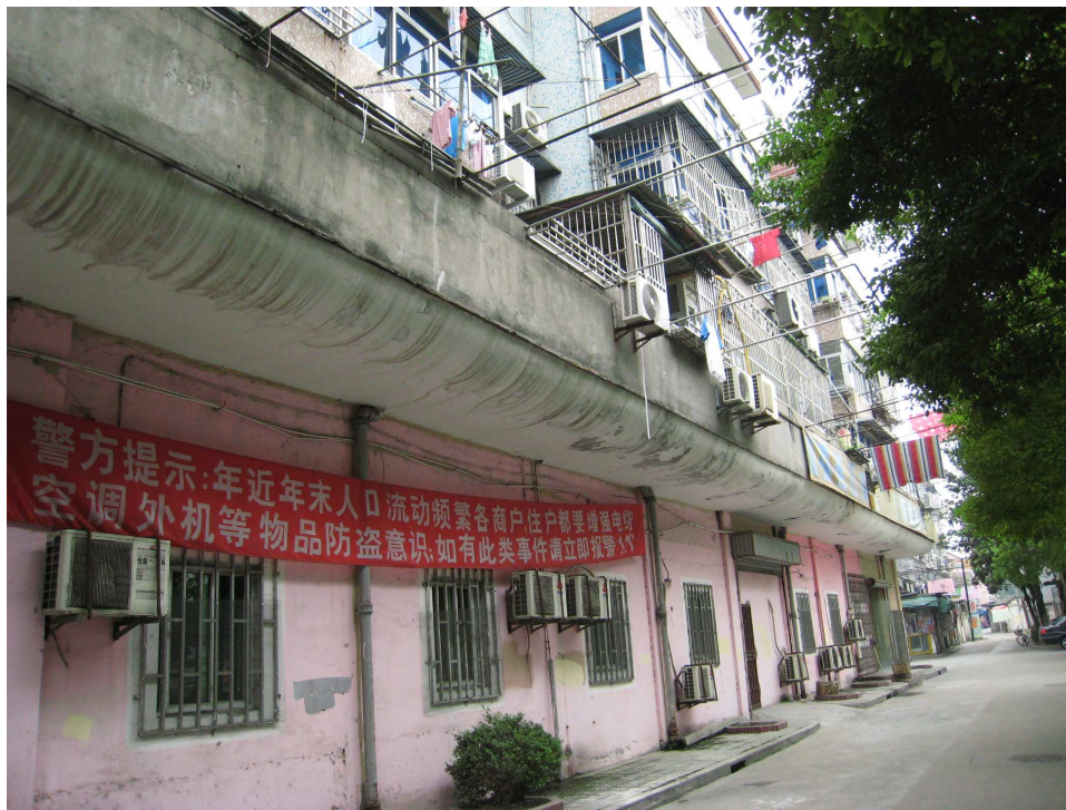
Figure 4-1. Warning Sign in an Urban Residential Area “Police Notice: Migrants Increased in Number before New Year, so please be Aware of Thefts of Properties such as External Parts of Air-Conditioners. Please report to the Police when you notice anyone
