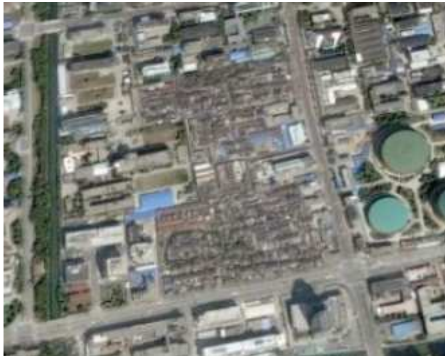
Figure 4-3. The Pond Community on Google Earth
