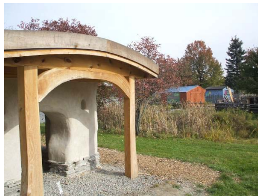
Figure 9: Straw bale "troll house" and wetland.
