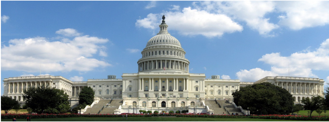
Figure 7: Front entrance view of the U.S. Capitol building
