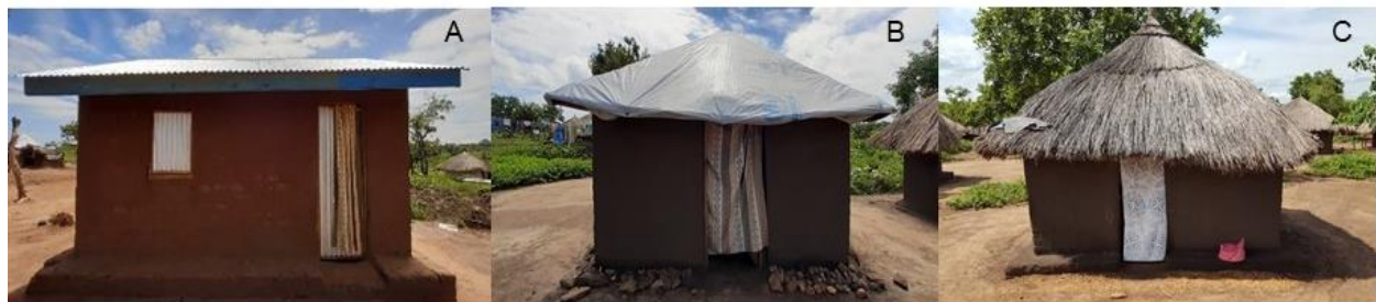
Figure 10. Photos of hut types from October 2020 pilot data collection. A) metal roof with window, B) tarp-covered roof, C) thatch roof.
