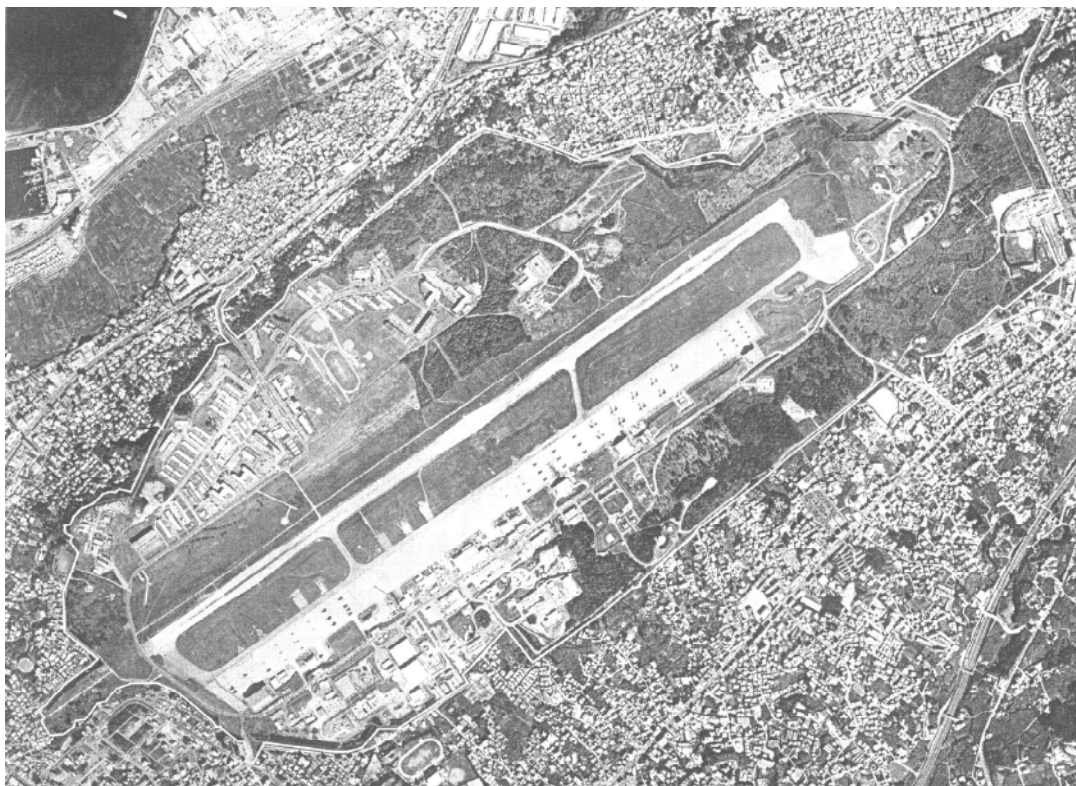
Figure 3.3: Aerial photo of Marine Corps Air Station Futenma, Ginowan City Source: MCAS Futenma Master Plan
