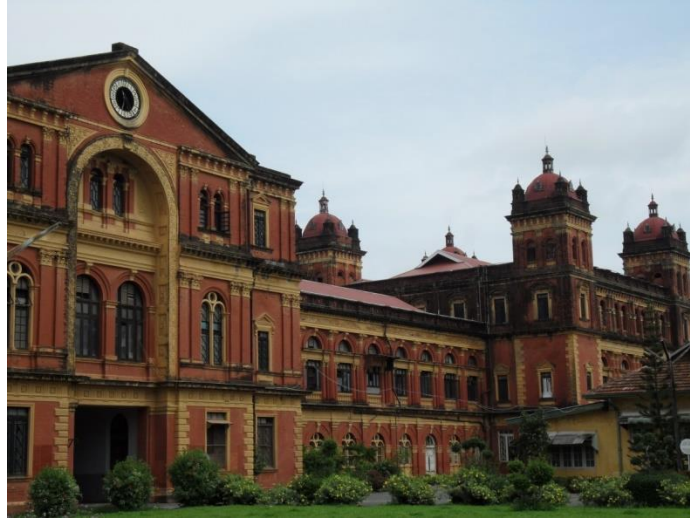
Figure 19. Secretariat (Minister's Building), Yangon. South elevation, looking west. (Credit: Author, 2012.)
