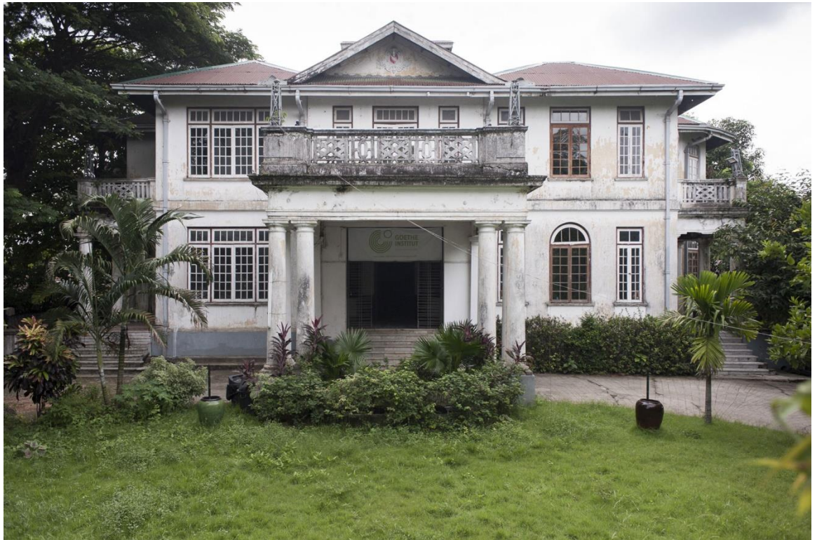
Figure 13: The home of the Goethe Institut Myanmar, prior to renovation. In this condition, it served as the setting for “Building Histories” in March 2015. (Credit: Goethe Institut Myanmar.)
