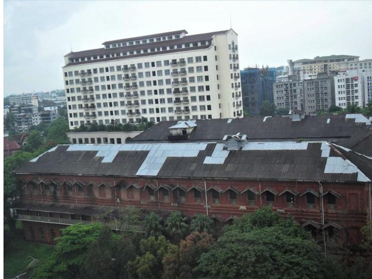
Figure 7. The Burma Railways Company Building, foreground, had been vacant since 1994 when it was purchased by a private company in exchange for the construction of new railway headquarters. ( Credit: Author, 2012. )
