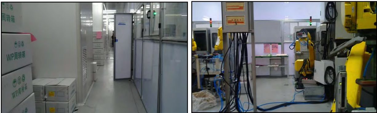
Above: machines and other items create potential fire escape hazards.
