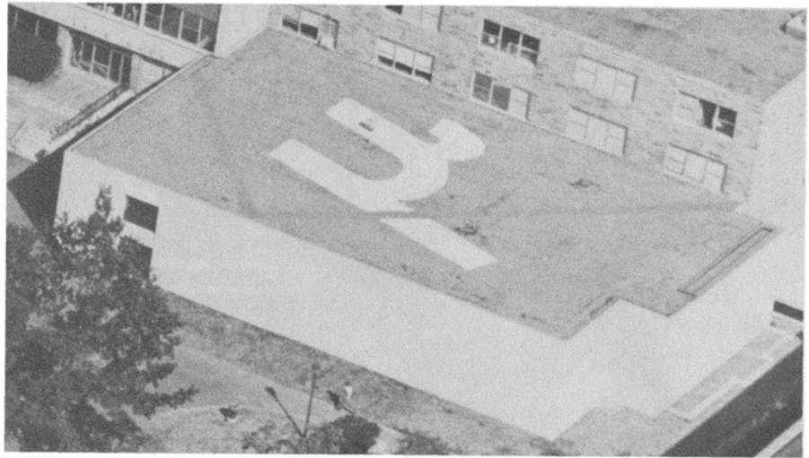
Colored gravel produces the symbols for 'less than' and 'micron' on the roof of the Submicron Facility, a wing on Phillips Hall, above.
