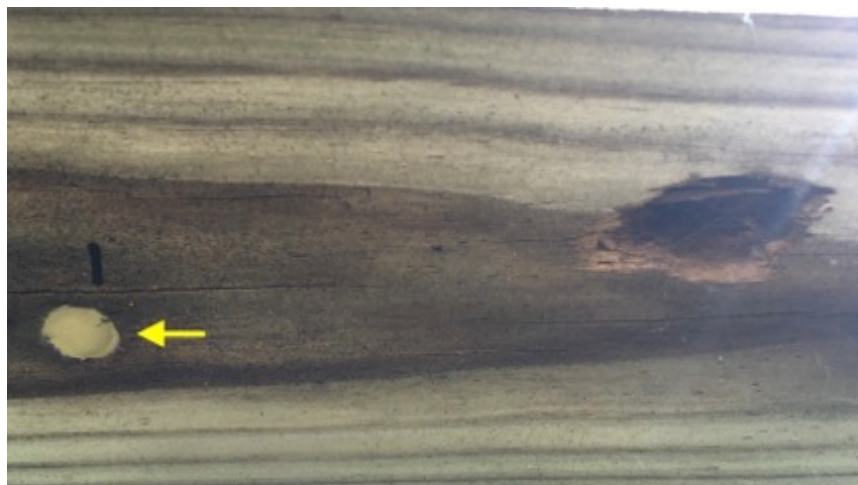
Fig. 2. Round openings created by carpenter bees (lower left) were sealed in this experiment, while holes created by woodpeckers (right) were not.
