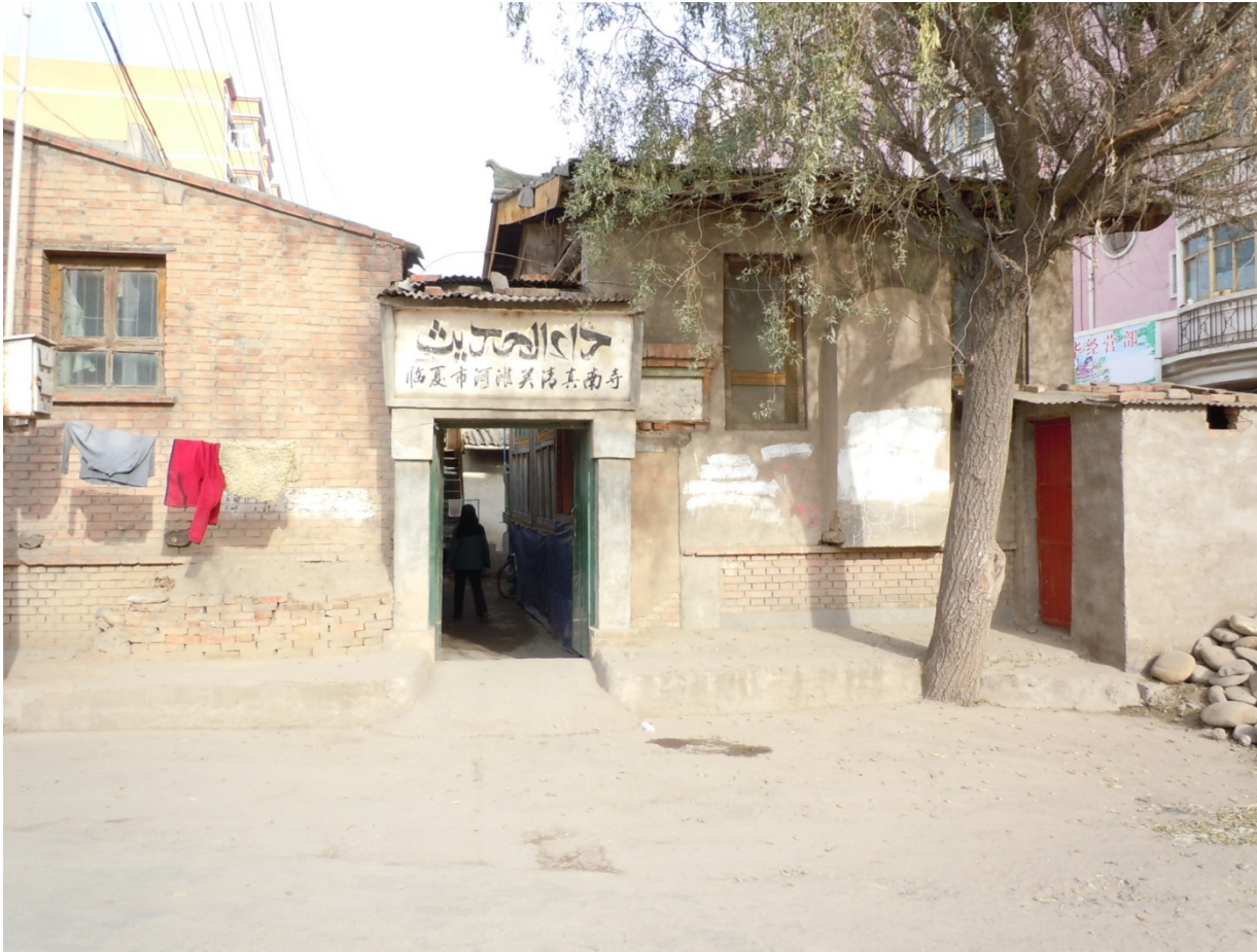
3.2. River Rapids South Mosque (11/7/2010).
