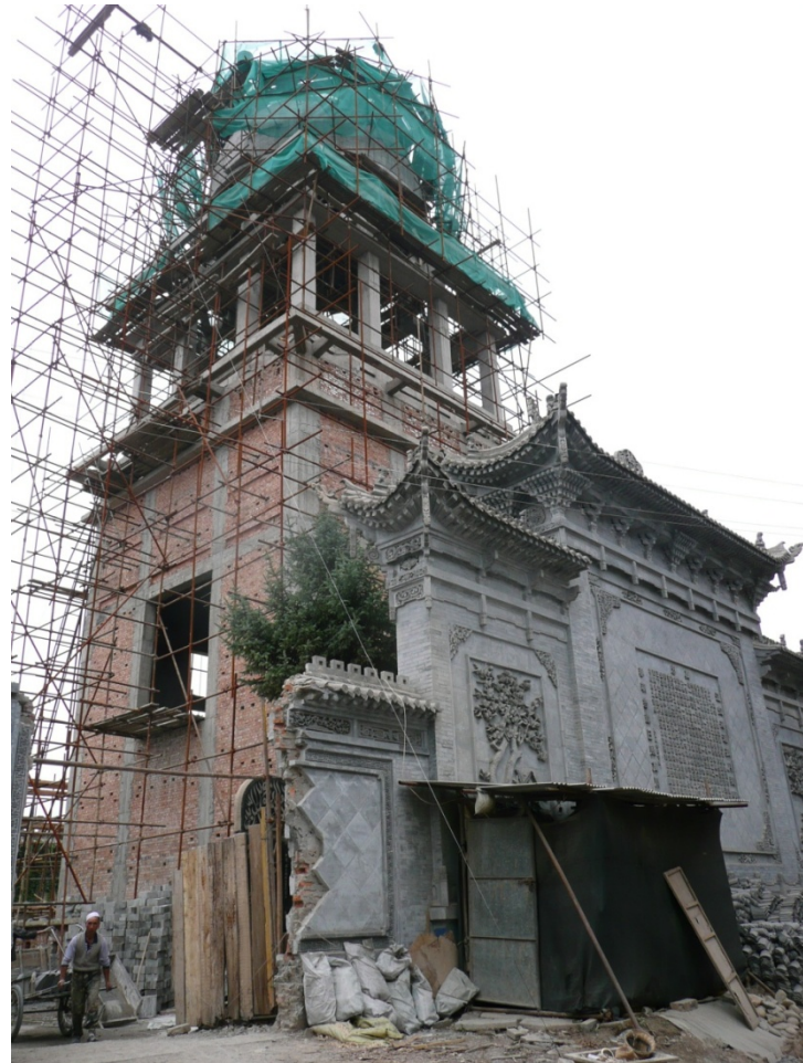
1.2. Guo Tomb Complex. Construction of tower (9/13/10).
