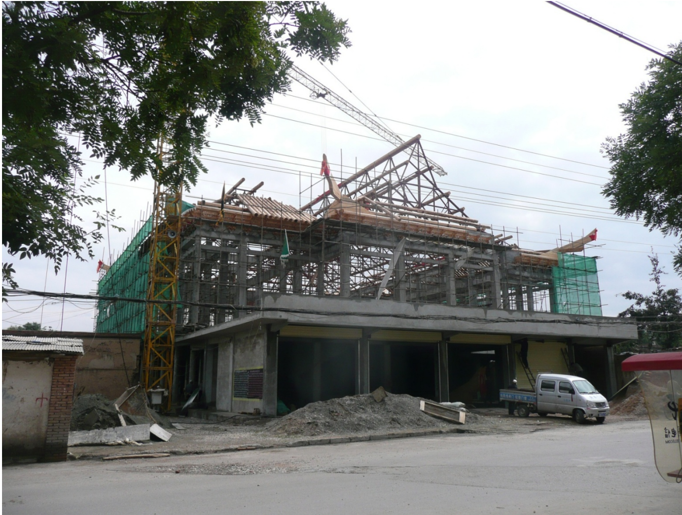
1.12. Constructing Bright Heart Mosque (12/17/2010).
