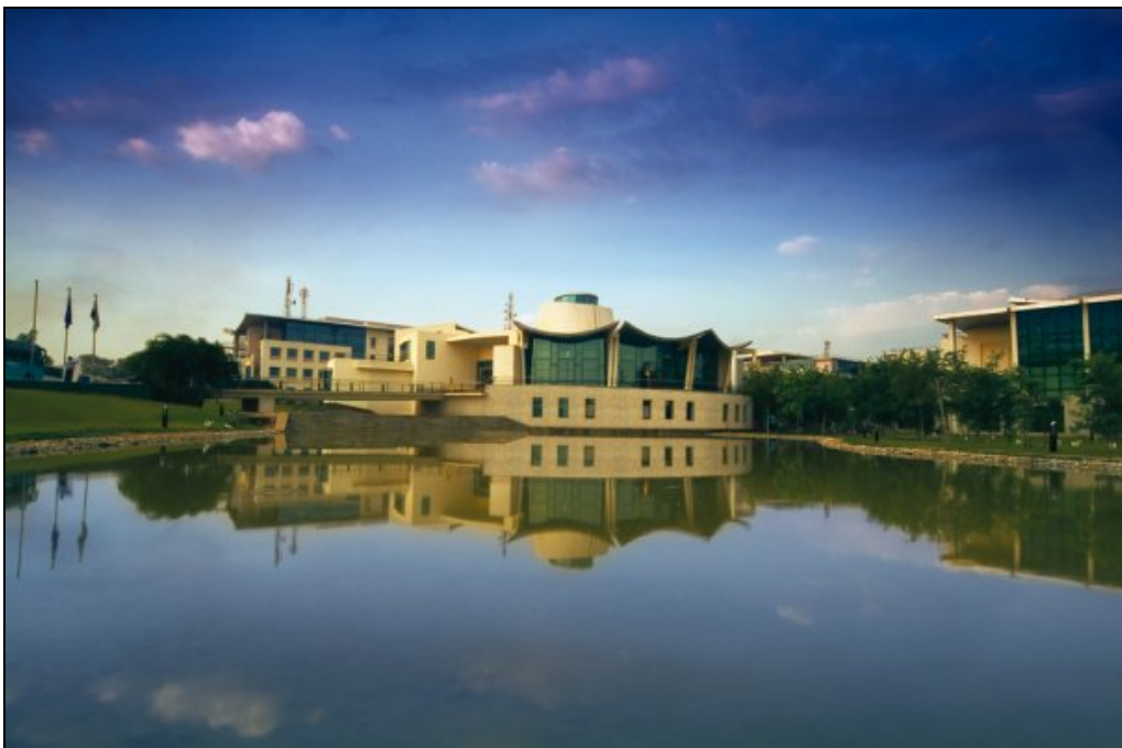
Figure 3.21-State-of-the art Learning Center Facility at Wipro's Electronics City Campus
