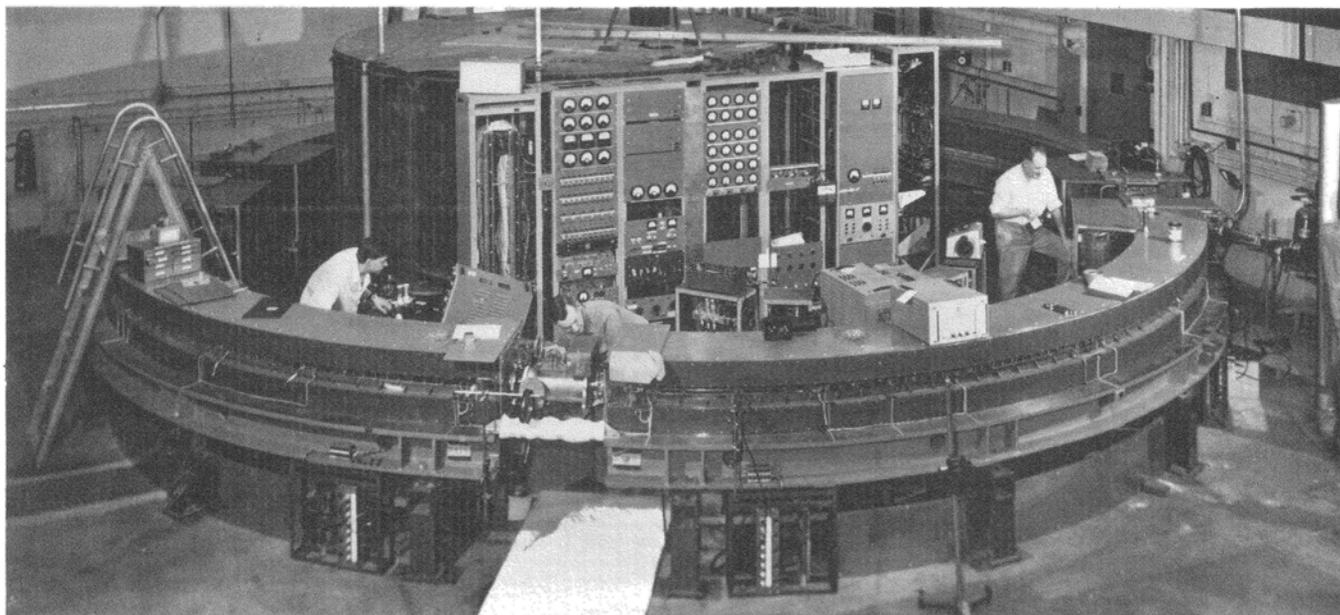
*The second and third Cornell accelerators sit one within the other in the Newman Lab in the 1960s. The second, a 300 MeV synchrotron, whirled electrons in an orbit of 6½-foot diameter, from 1949-53. The third, about 30 feet across, operated at a maximum level of 1.4 GeV, from 1960-65. A fourth, 2 GeV synchrotron replaced it for the three years before today's 10-GeV one went into operation under Alumni Field in 1968.*
