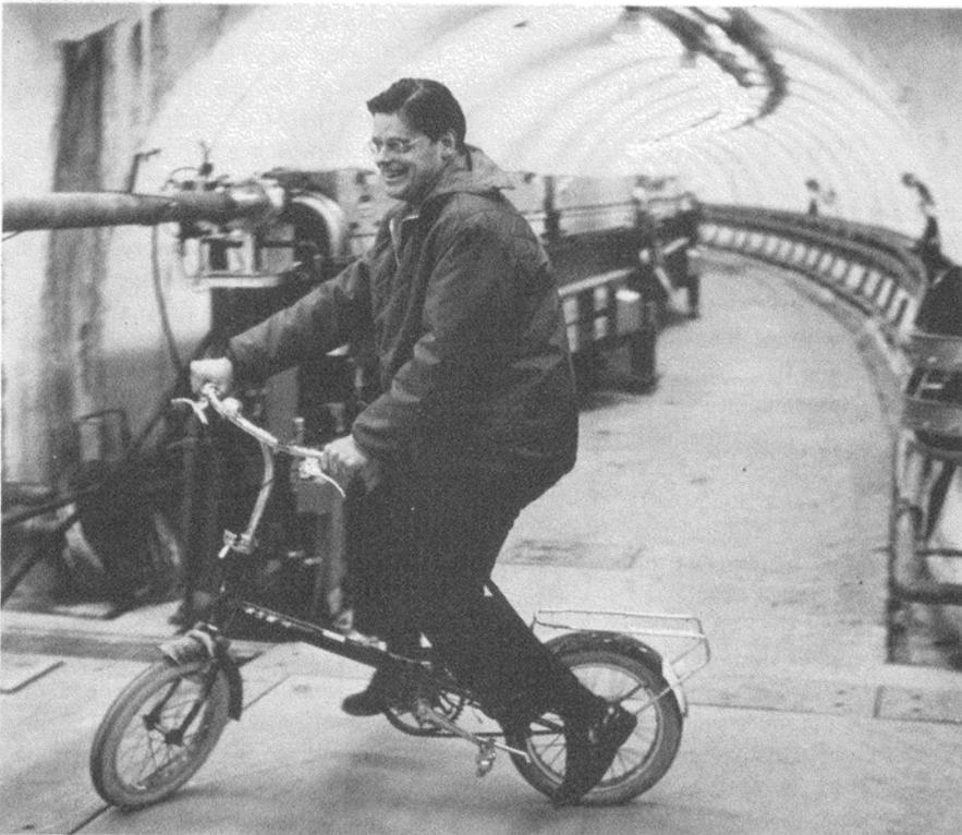
*Synchrotron beam chamber emerges from the tunnel at left into hall where particle collisions occur and are recorded. At left, Prof. Robert Wilson, first director, for whom the lab is named, uses a bicycle to travel the new beam tunnel in 1967. A second beam ring has since been added against the tunnel's outside wall, increasing the energy available to the interactions to 16 GeV.*
