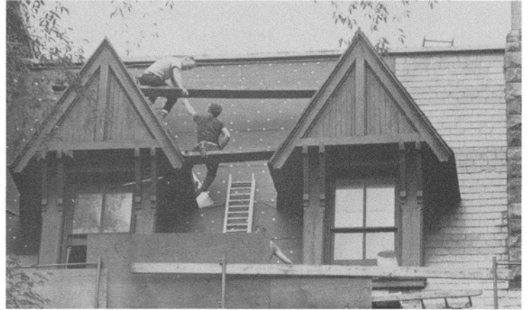
Workmen place tiles on mansard roof of Franklin.—Gray '71
