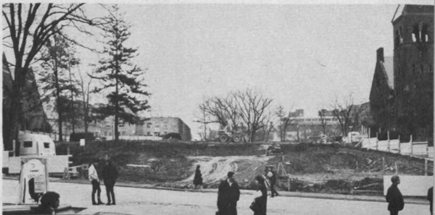
Digging opens way for underground campus store.
