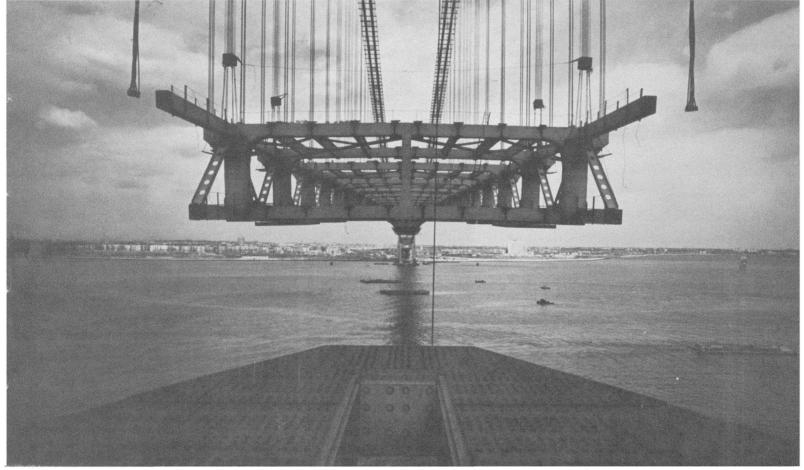
By March 1964, deck platforms for the bridge reach out to join Brooklyn and Staten Island. Deck hangs from cables.
